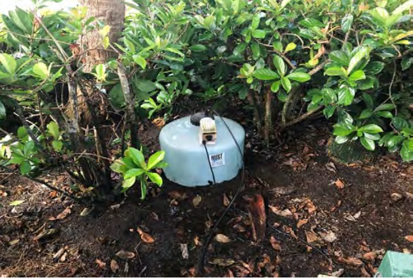
Irrigation Expansion Tank
