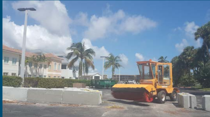
1000 North making progress with building construction and about to start parking lot upgrades.
