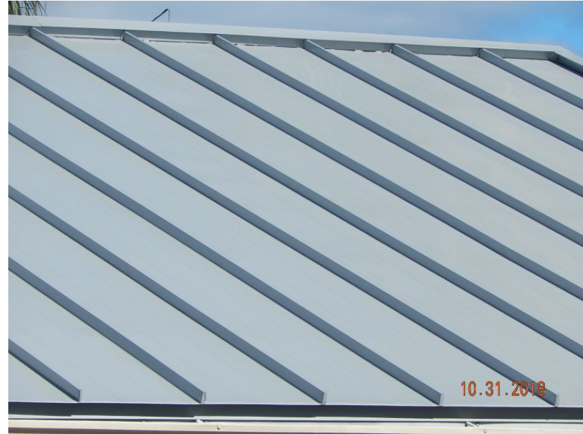
Metal Roof Covering
