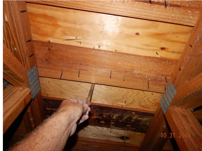
1/2" Deck Thickness Confirmed
