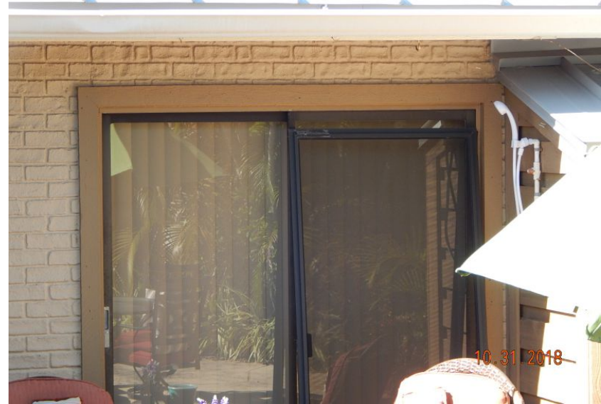
Unprotected Glazed Entry Door
