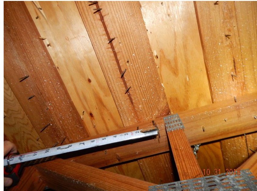
Plywood Over Battens
