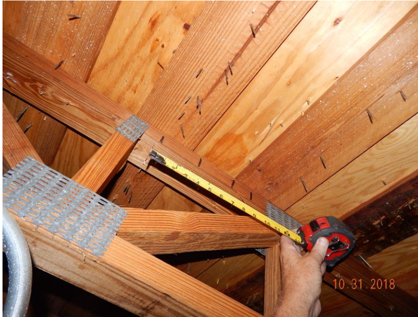
Plywood Over Battens
