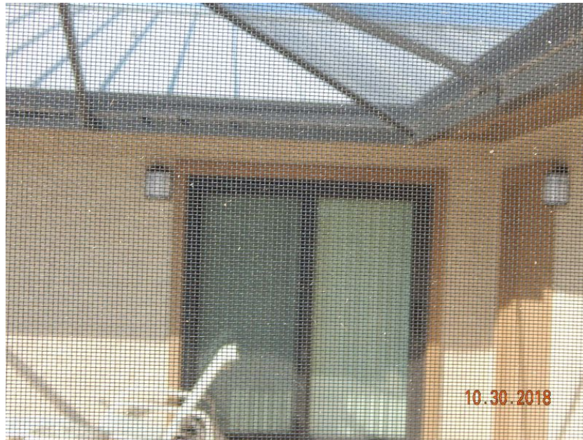
Unprotected Glazed Entry Door
