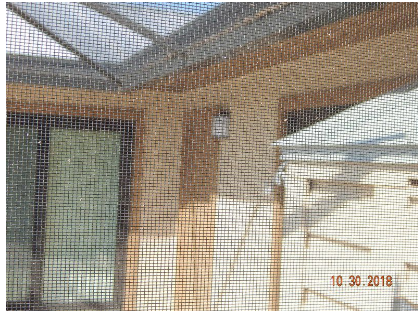
Unprotected Solid Entry Door
