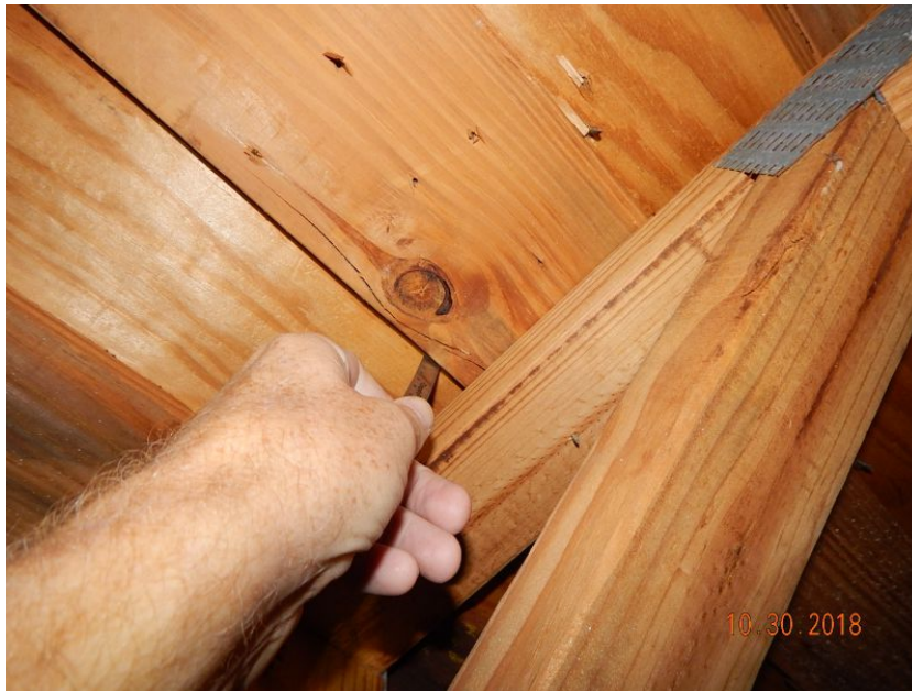
1/2" Deck Thickness Confirmed
