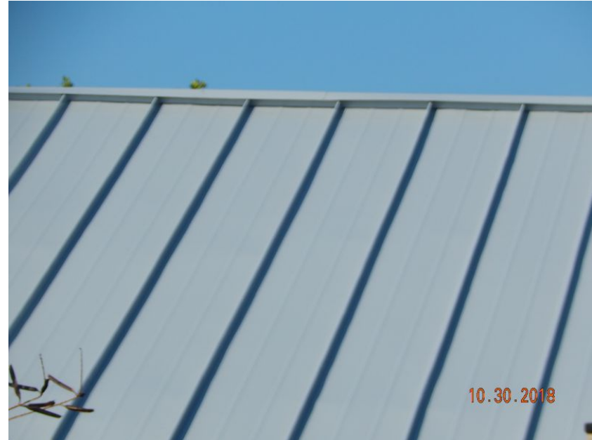
Metal Roof Covering
