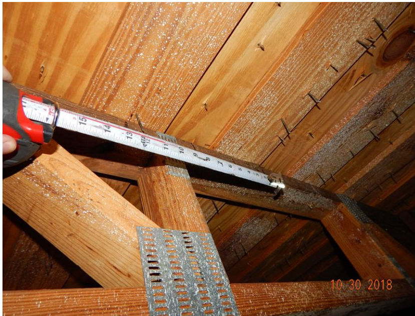
Plywood Over Battens
