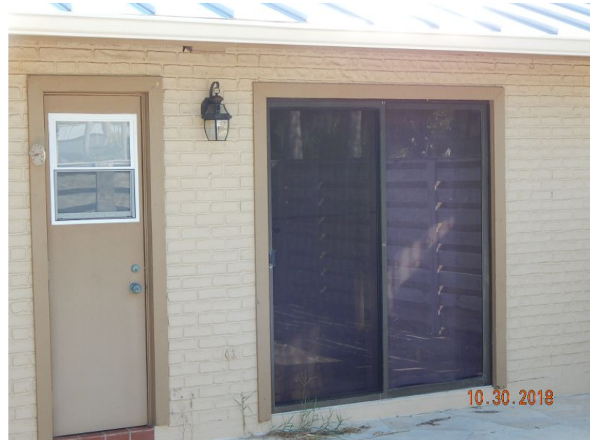
Unprotected Glazed Entry Door
