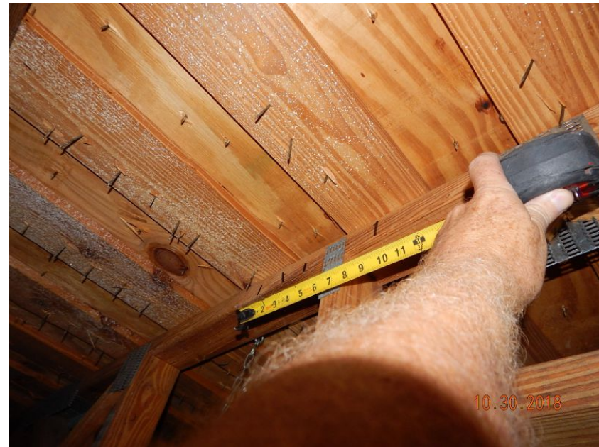
Plywood Over Battens
