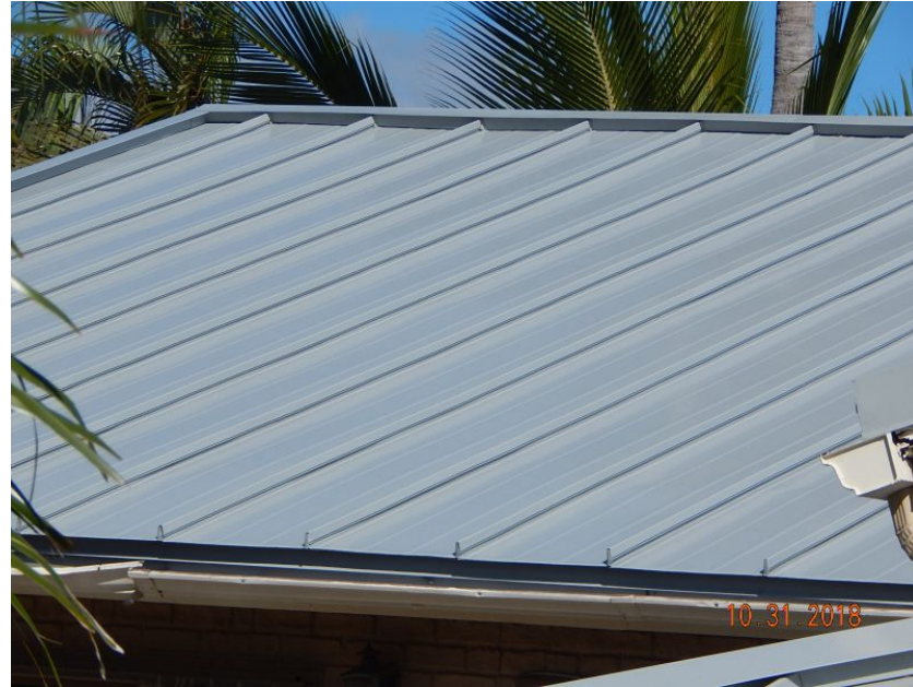
Metal Roof Covering
