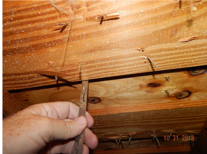
1/2" Deck Thickness Confirmed
