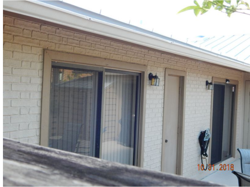
Unprotected Glazed Entry Door
