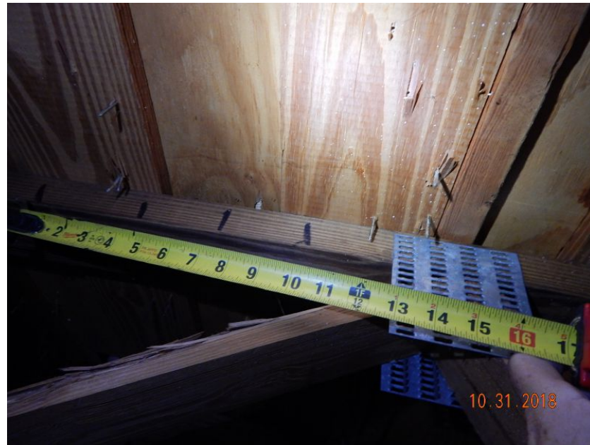
Plywood Over Battens
