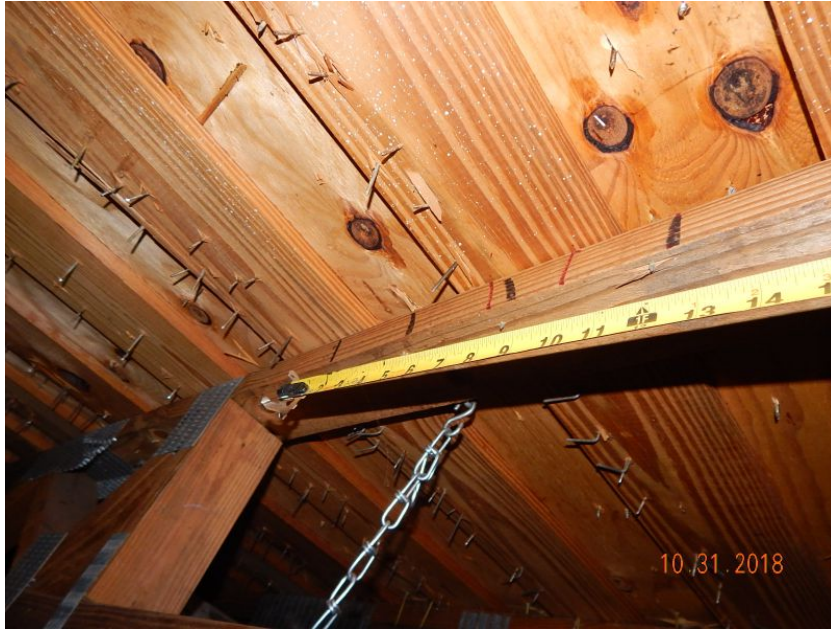
Plywood Over Battens
