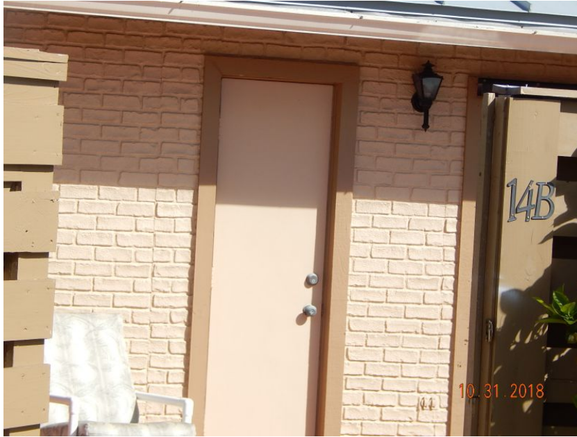
Unprotected Solid Entry Door
