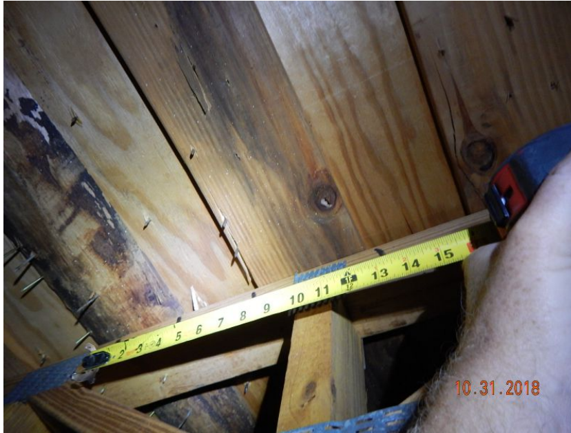
Plywood Over Battens
