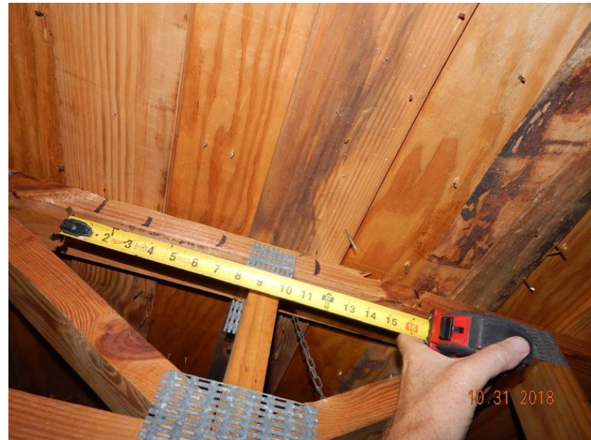
Plywood Over Battens
