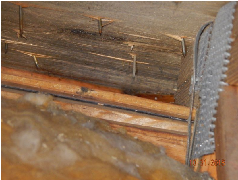
Metal Connector with 1 Nail on Each Side
