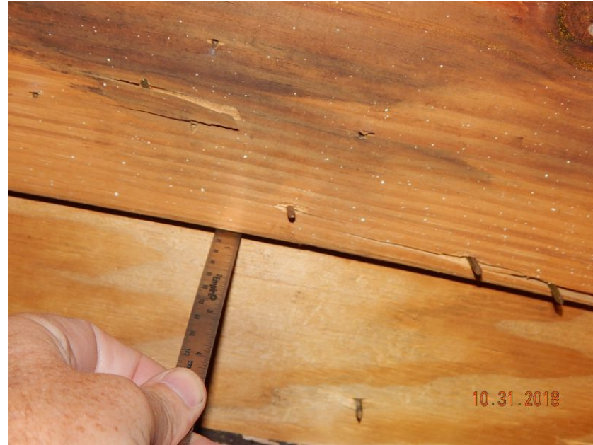
1/2" Deck Thickness Confirmed
