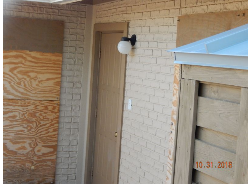
Unprotected Solid Entry Door
