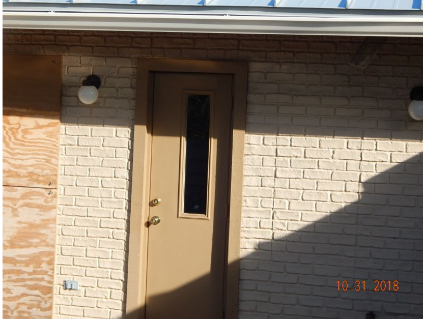
Unprotected Glazed Entry Door
