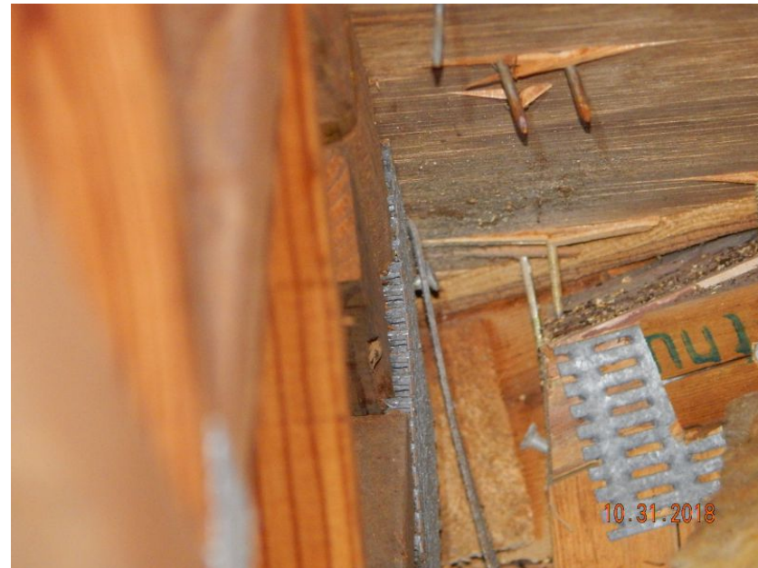
Metal Connector with 1 Nail on Each Side
