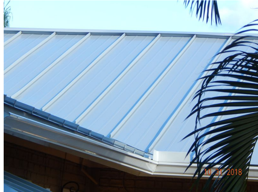
Metal Roof Covering
