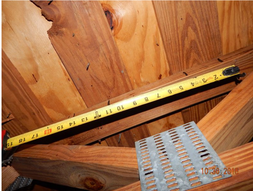
Plywood Over Battens
