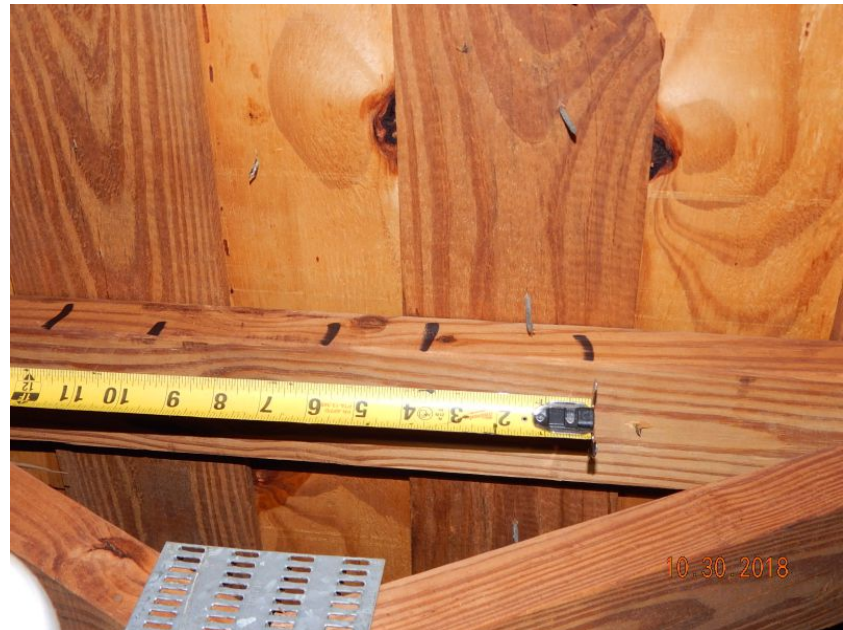
Plywood Over Battens
