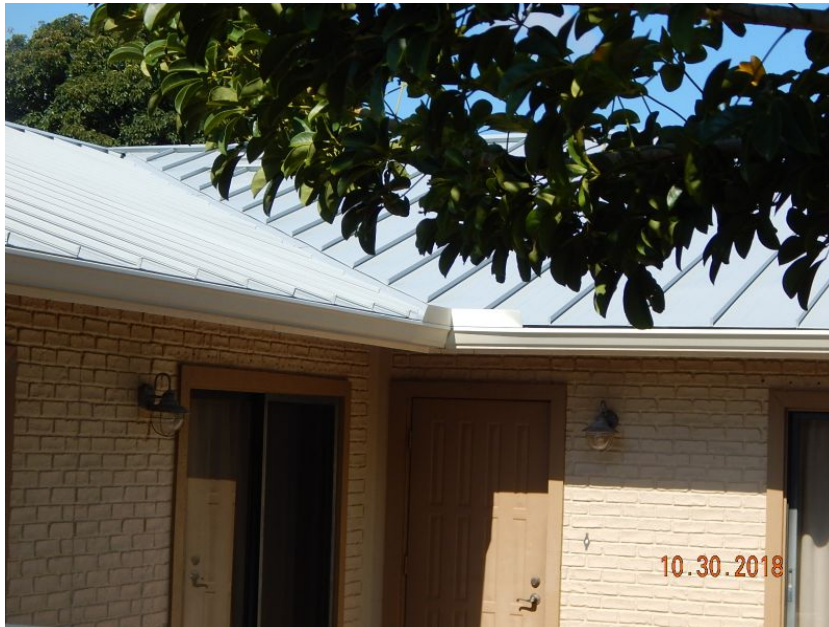
Unprotected Glazed Entry Door
