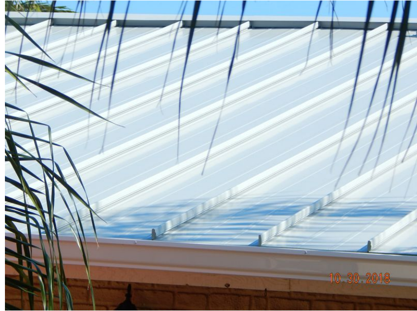
Metal Roof Covering
