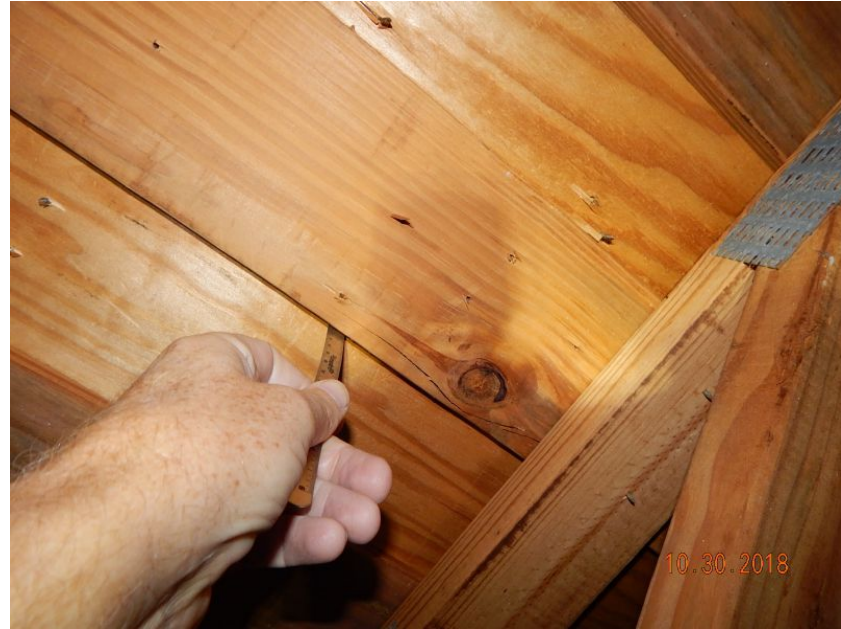
19/32" Deck Thickness Confirmed
