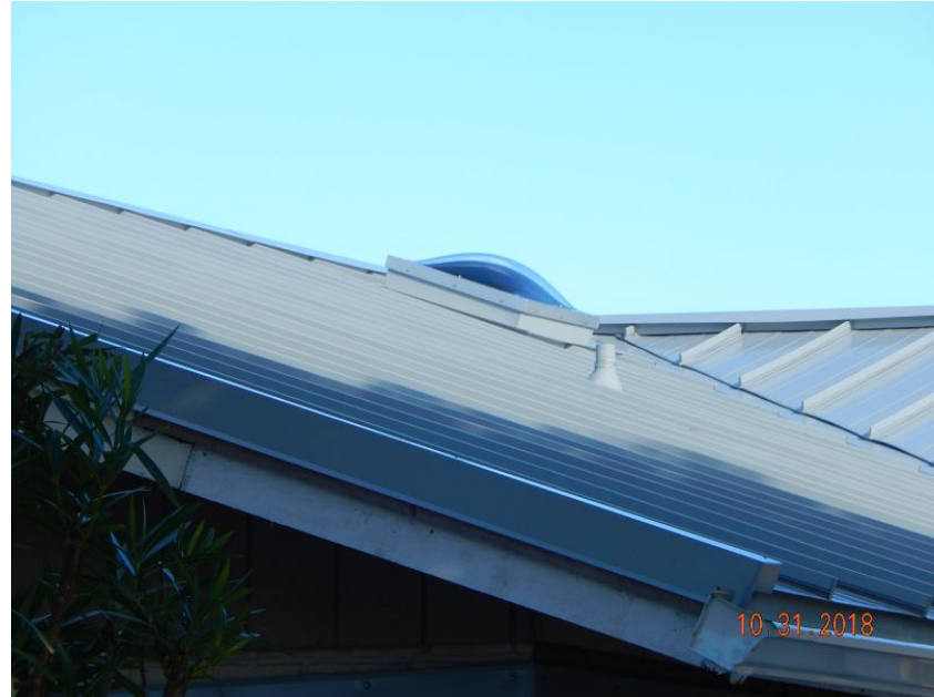
Metal Roof Covering
