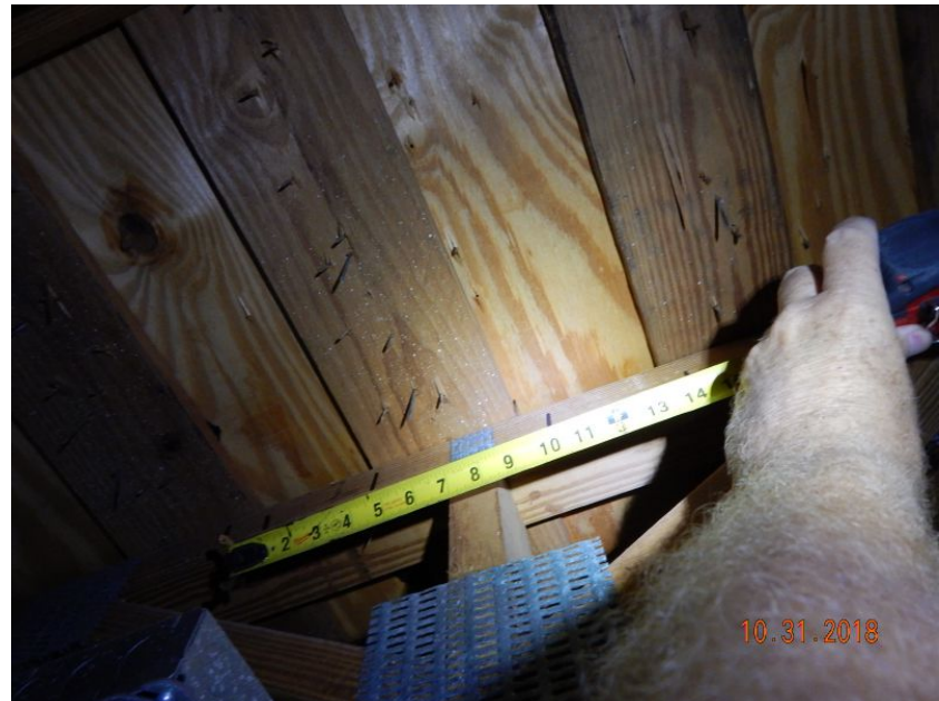
Plywood Over Battens
