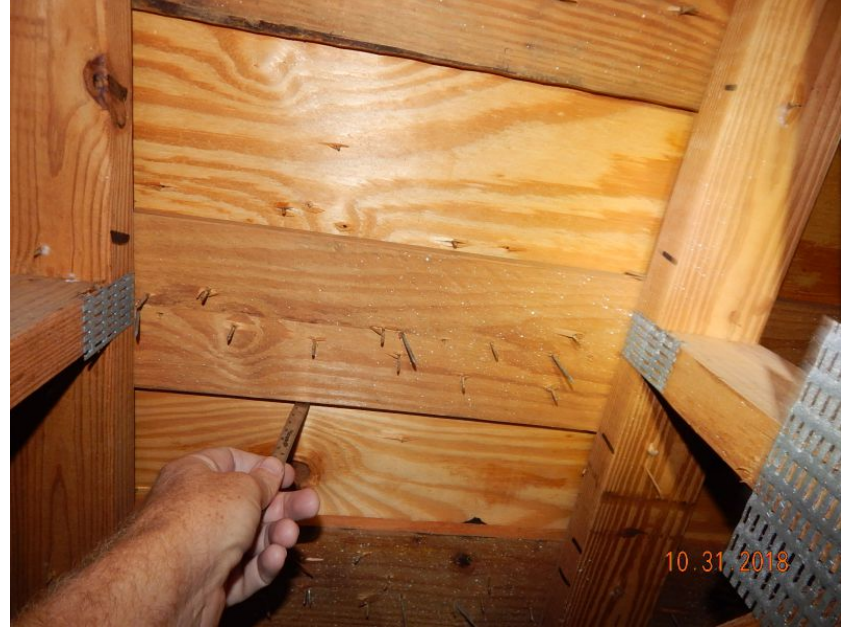
1/2" Deck Thickness Confirmed
