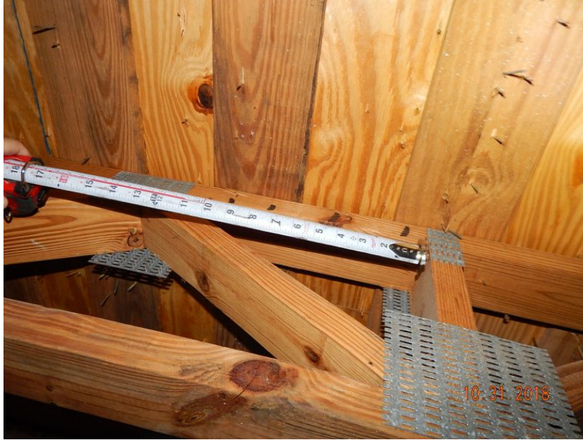
Plywood Over Battens
