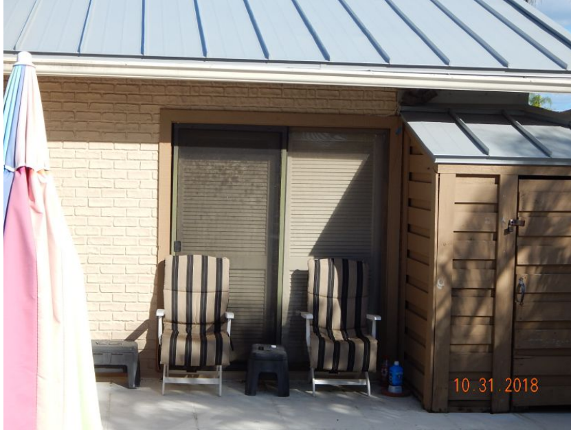
Unprotected Glazed Entry Door
