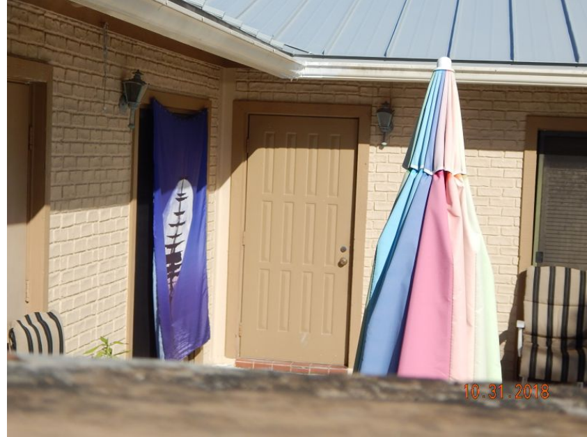
Unprotected Solid Entry Door
