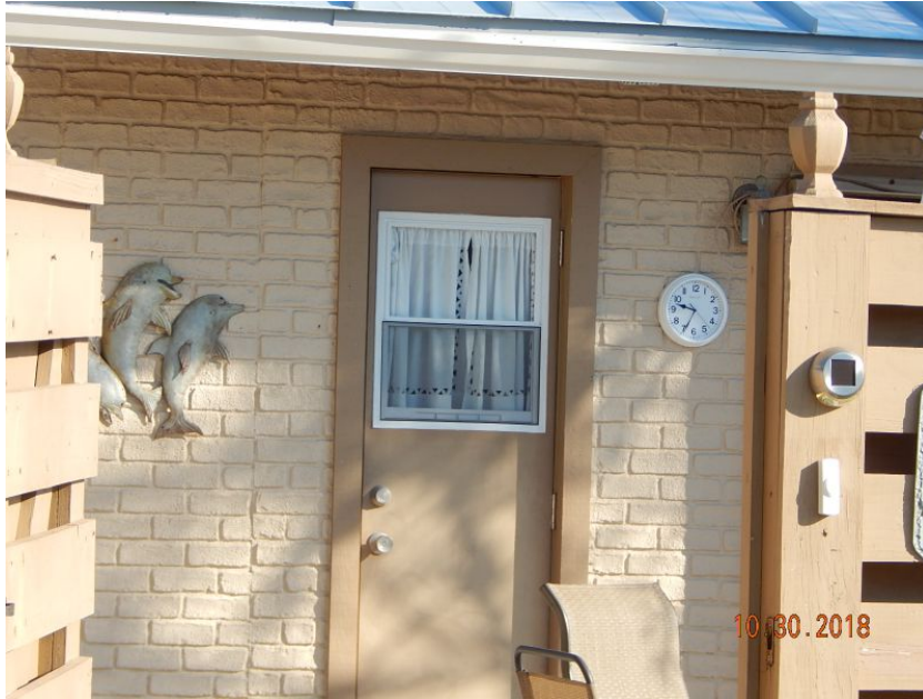
Unprotected Glazed Entry Door
