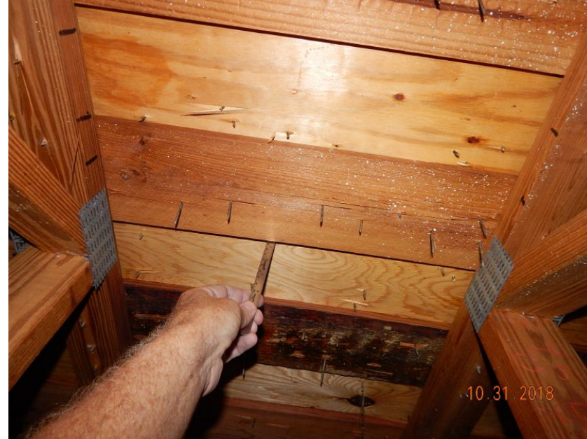
1/2" Deck Thickness Confirmed
