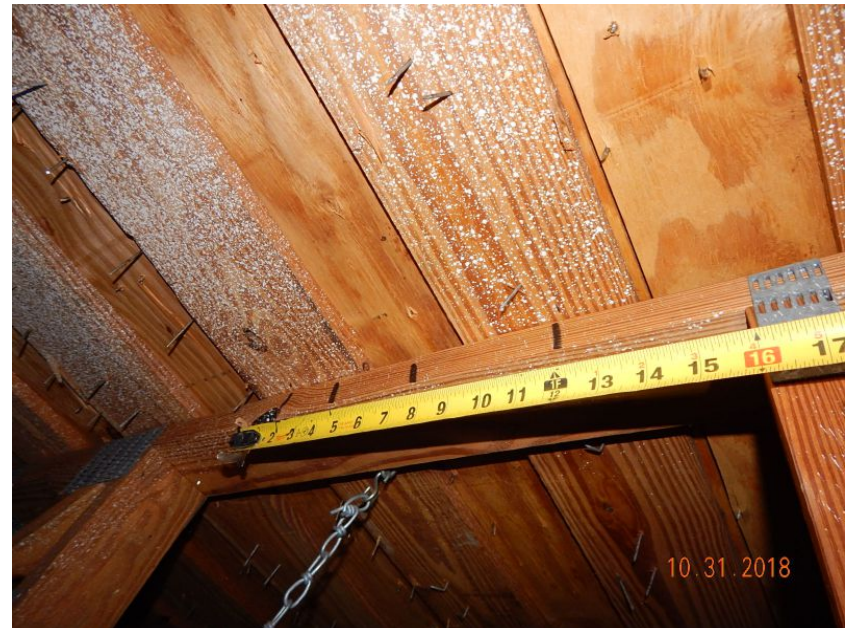
Plywood Over Battens
