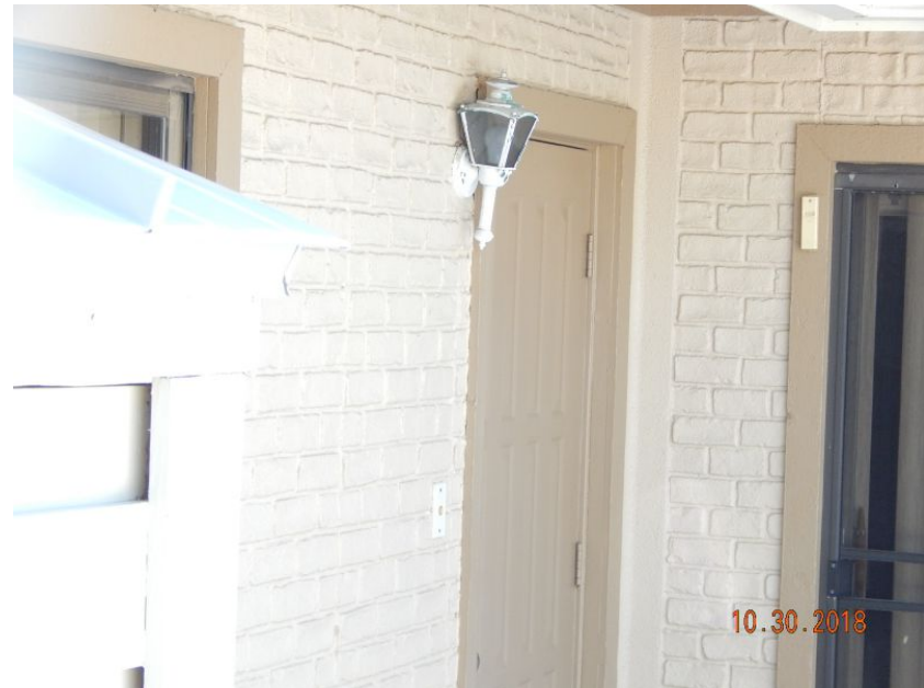
Unprotected Solid Entry Door
