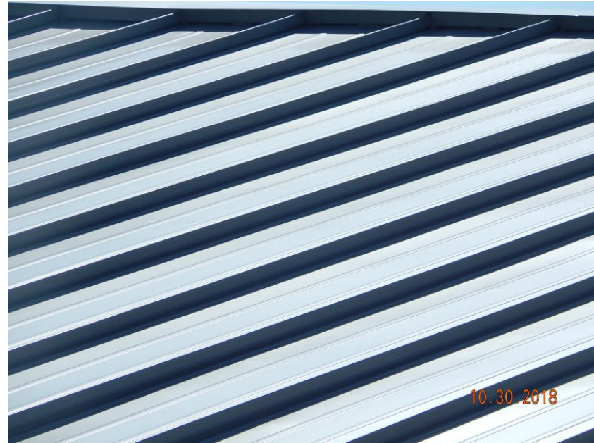
Metal Roof Covering
