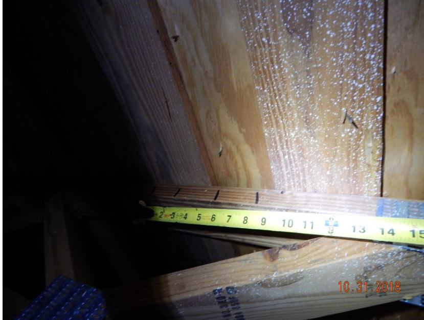
Plywood Over Battens
