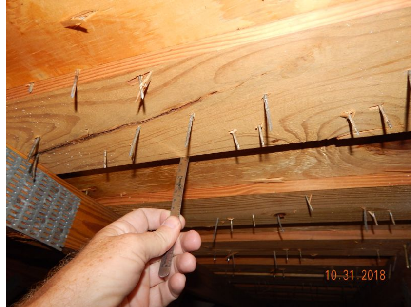
1/2" Deck Thickness Confirmed
