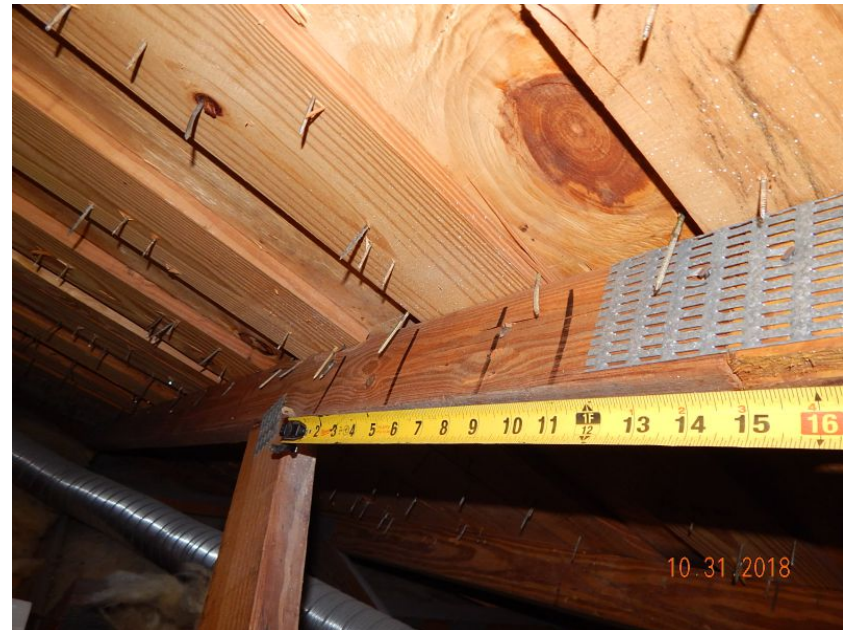
Plywood Over Battens
