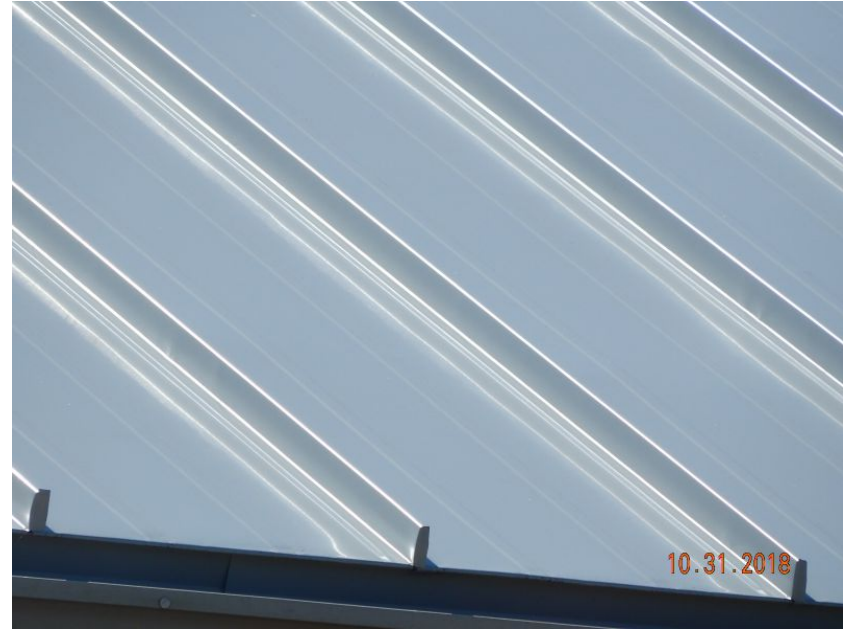
Metal Roof Covering
