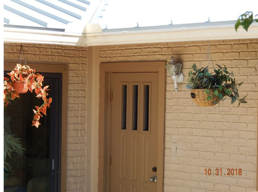
Unprotected Glazed Entry Door
