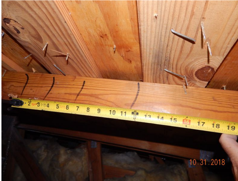
Plywood Over Battens
