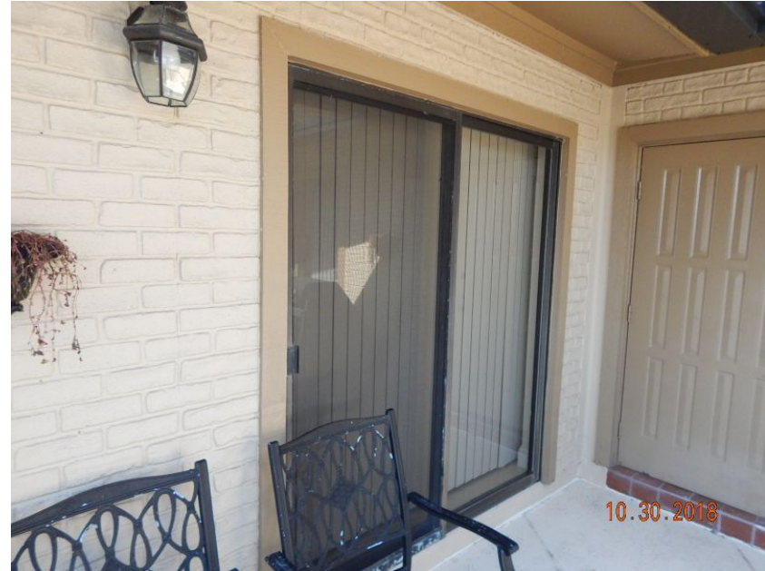
Unprotected Glazed Entry Door
