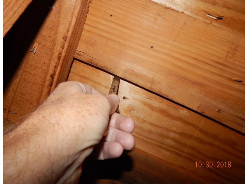
1/2" Deck Thickness Confirmed
