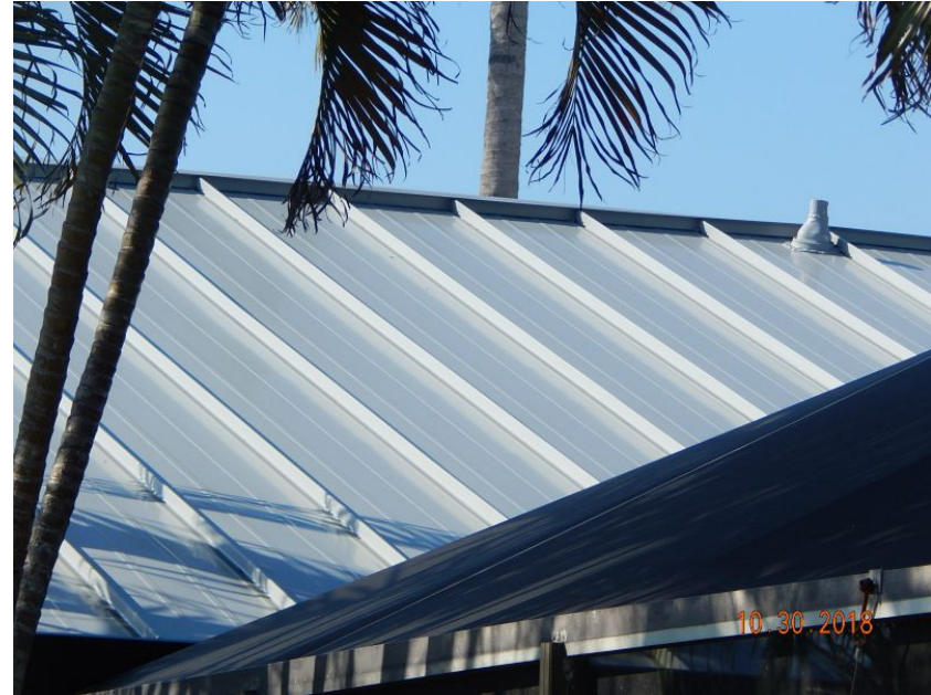
Metal Roof Covering
