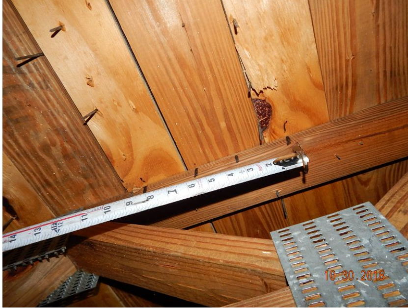
Plywood Over Battens
