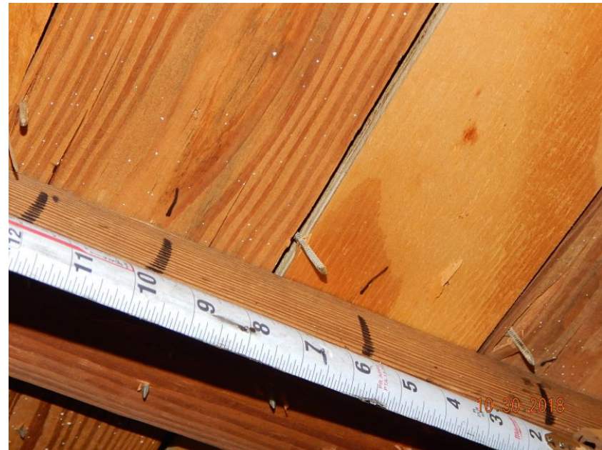
Plywood Over Battens
