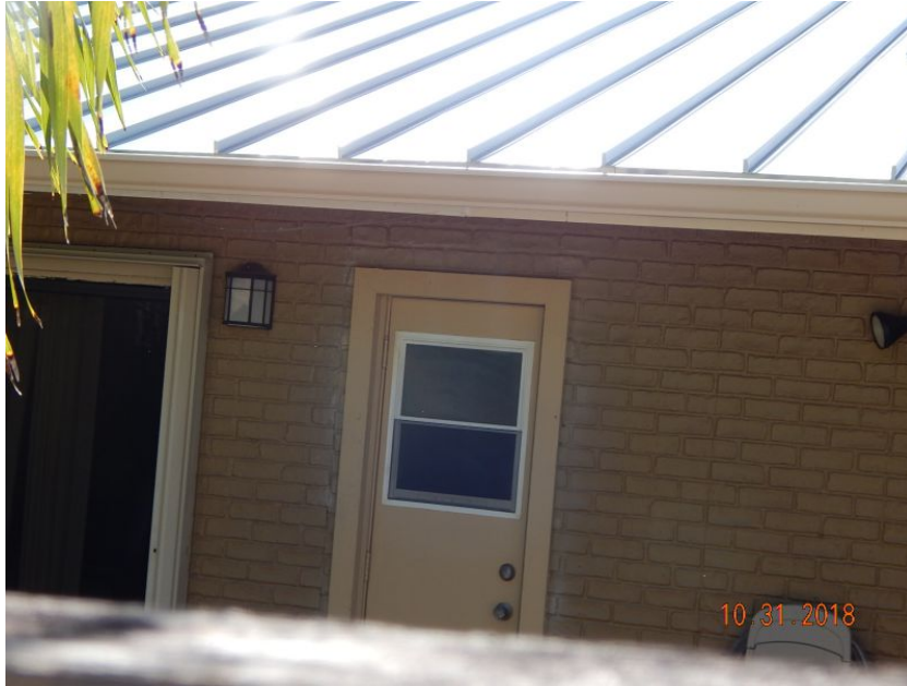
Unprotected Glazed Entry Door
