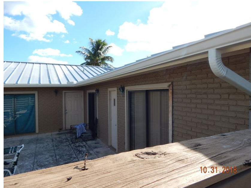
Unprotected Glazed Entry Door
