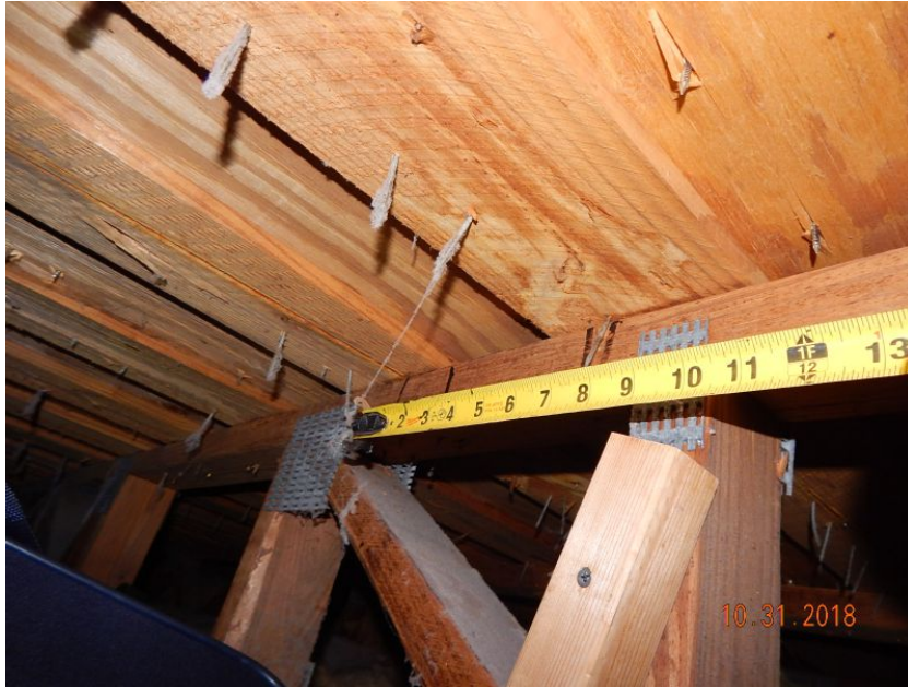
Plywood Over Battens
