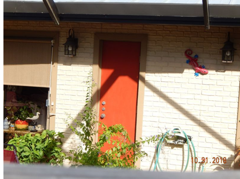
Unprotected Solid Entry Door
