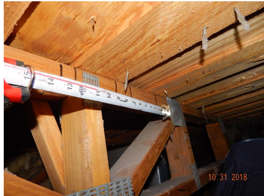
Plywood Over Battens
