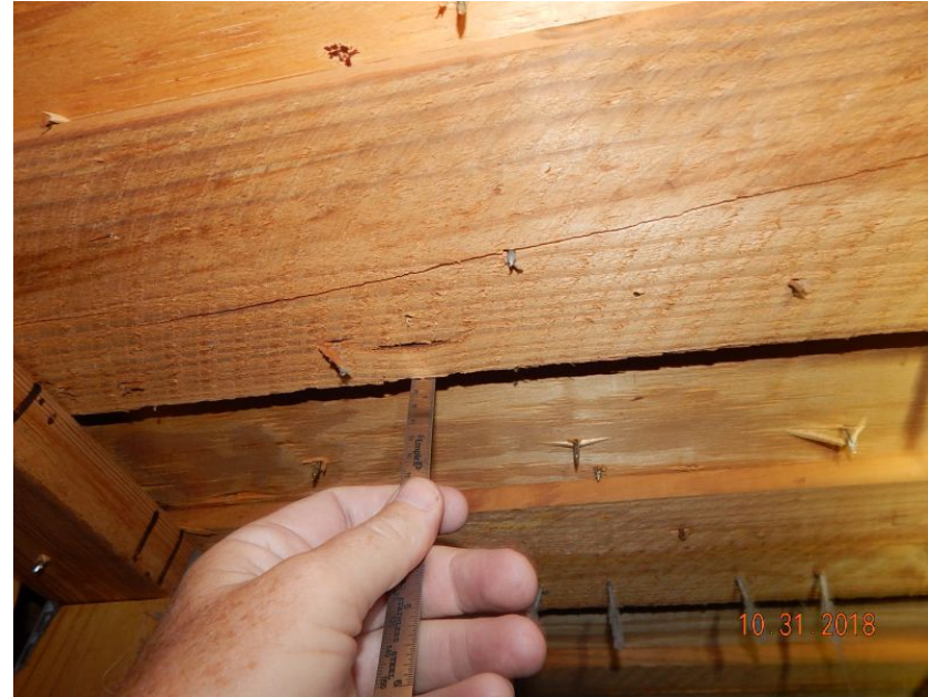
1/2" Deck Thickness Confirmed
