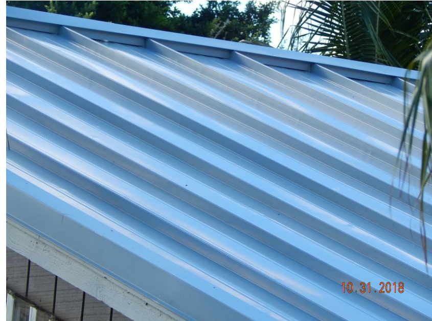
Metal Roof Covering
