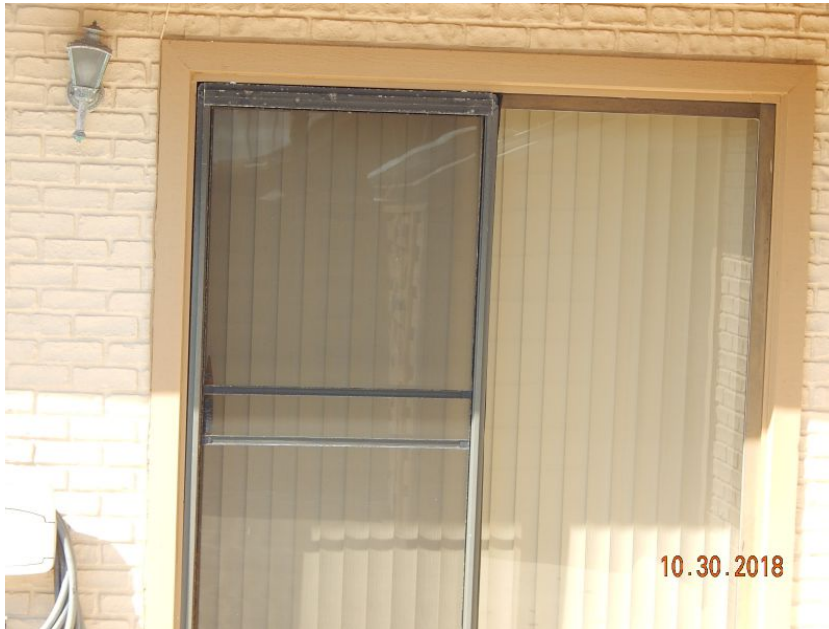
Unprotected Glazed Entry Door
