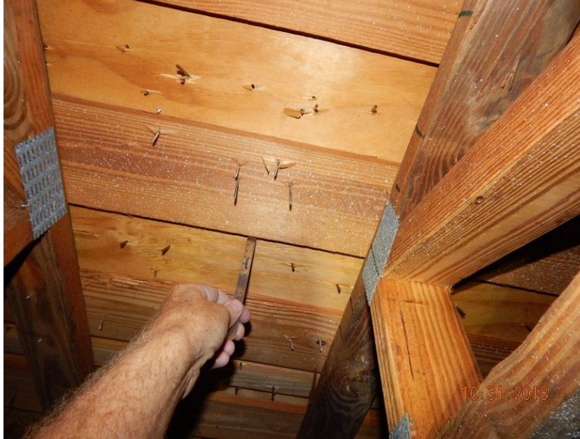
1/2" Deck Thickness Confirmed
