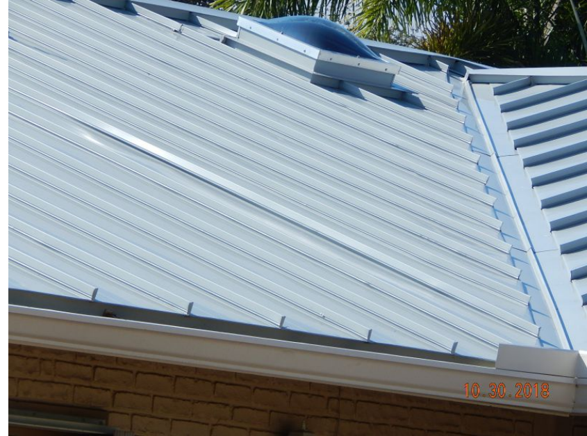
Metal Roof Covering
