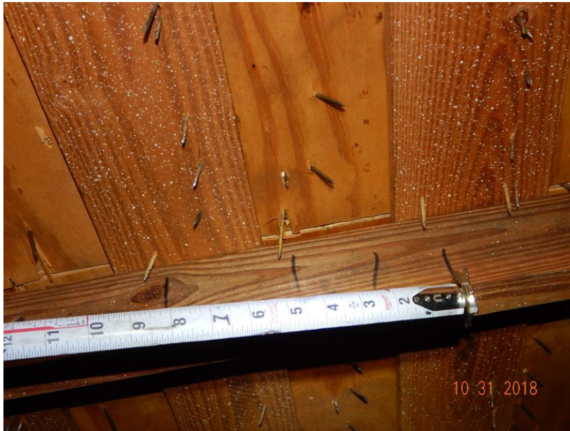
Plywood Over Battens
