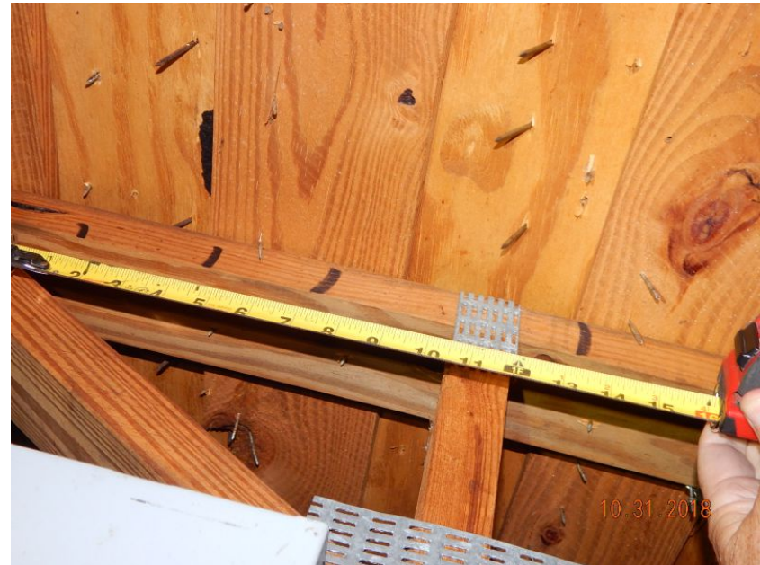
Plywood Over Battens
