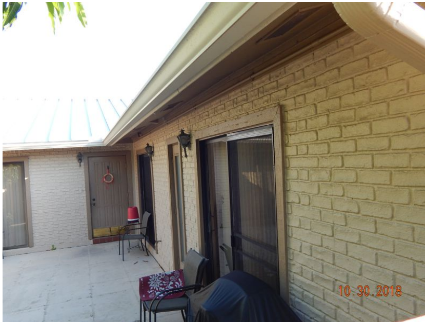
Unprotected Glazed Entry Door
