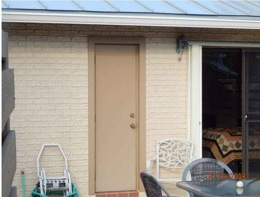
Unprotected Solid Entry Door
