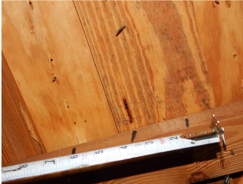
Plywood Over Battens
