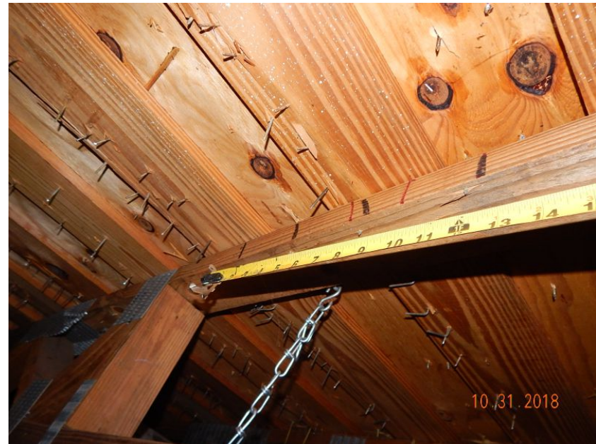
1/2" Deck Thickness Confirmed
