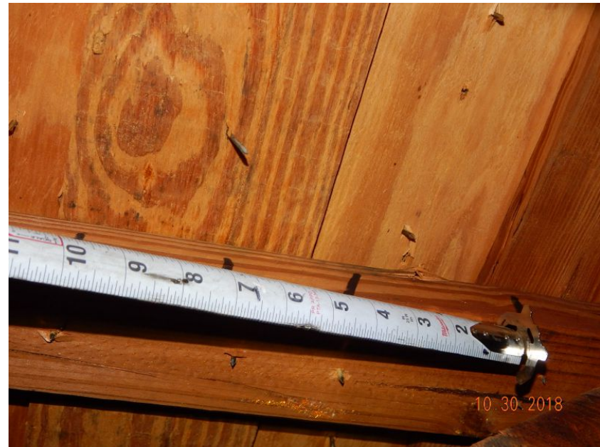
Plywood Over Battens
