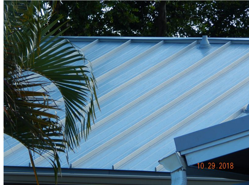
Metal Roof Covering
