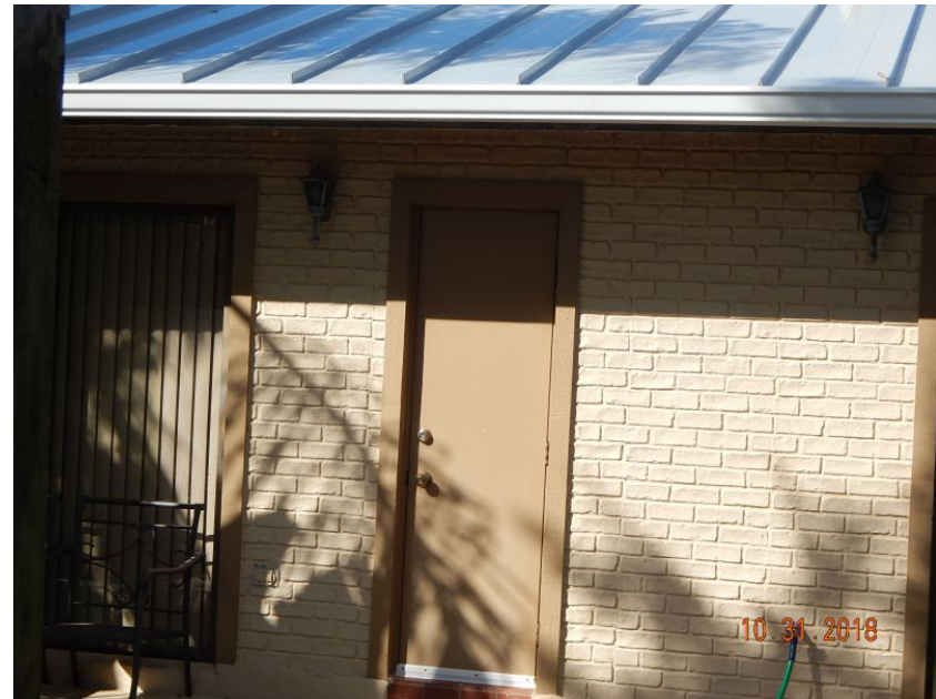
Unprotected Solid Entry Door
