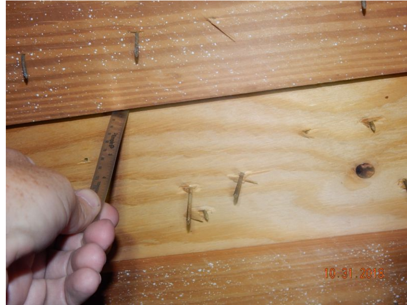
1/2" Deck Thickness Confirmed
