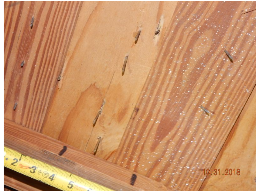
Plywood Over Battens
