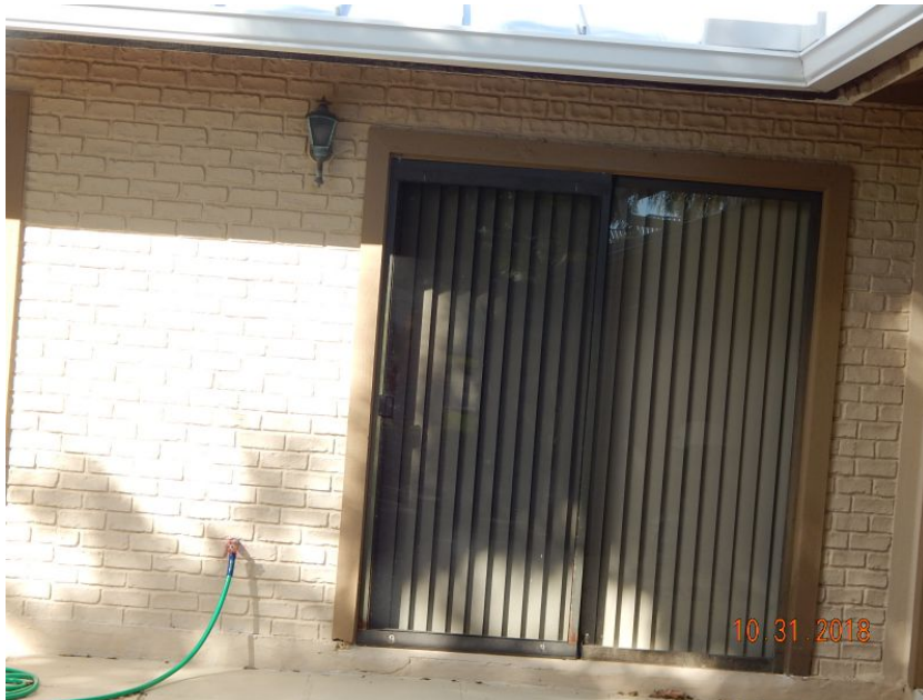
Unprotected Glazed Entry Door
