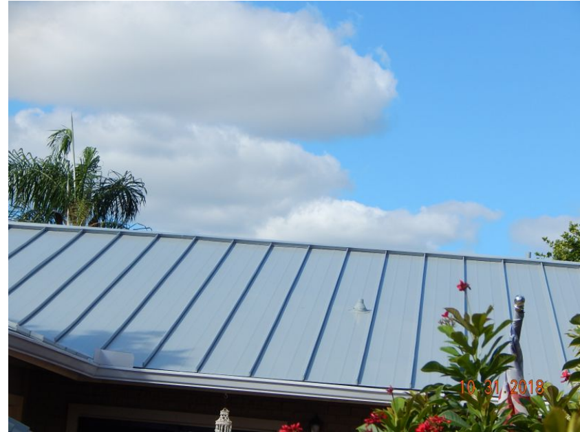
Metal Roof Covering
