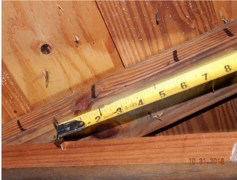
Plywood Over Battens
