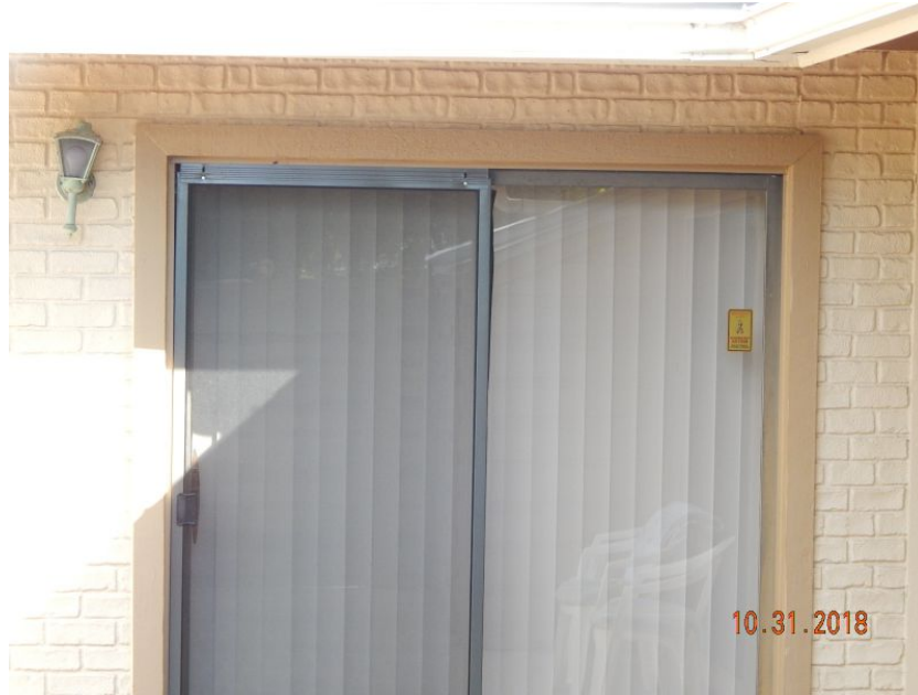
Unprotected Glazed Entry Door
