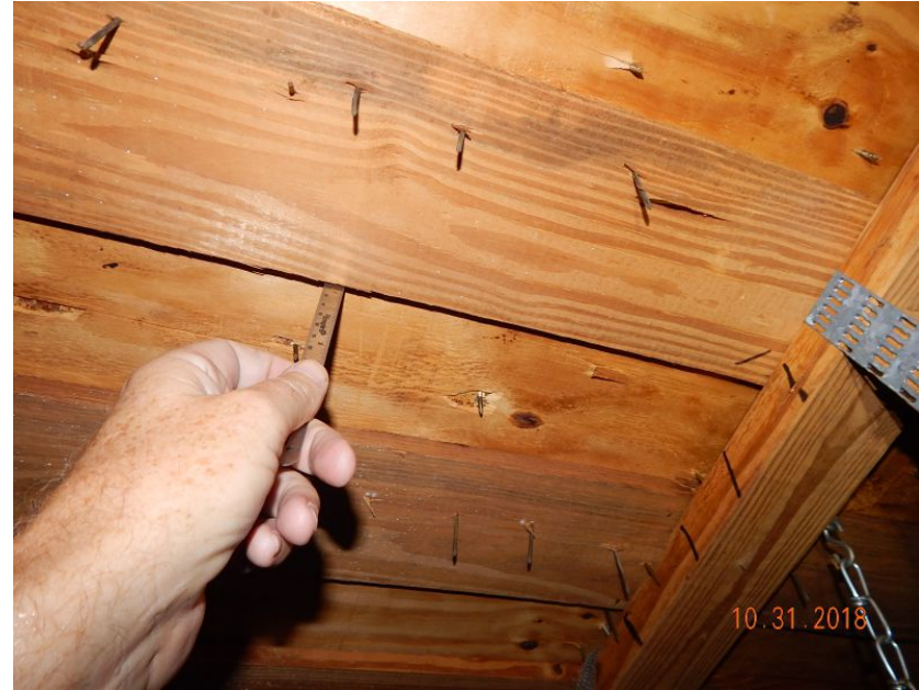
1/2" Deck Thickness Confirmed
