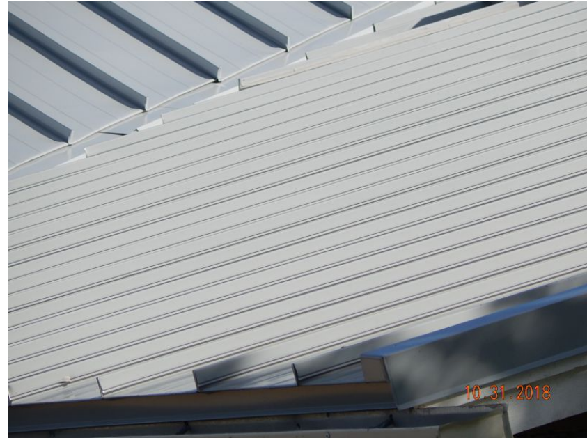
Metal Roof Covering
