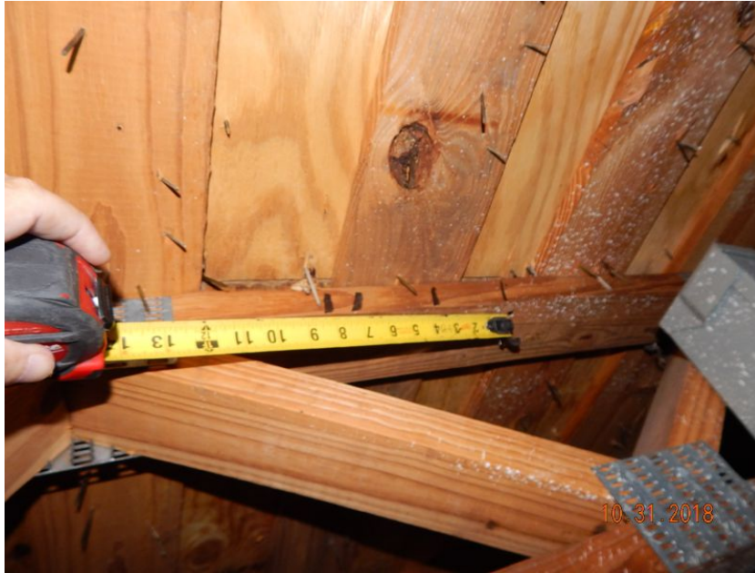
Plywood Over Battens
