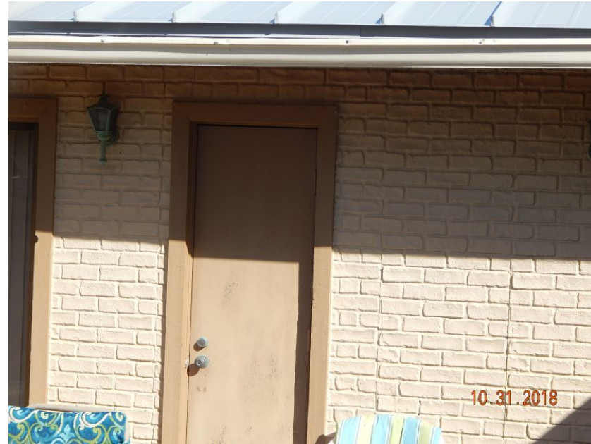
Unprotected Solid Entry Door
