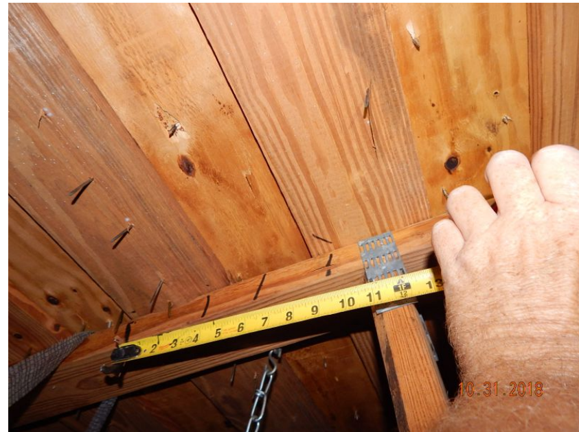
Plywood Over Battens
