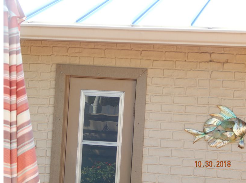
Unprotected Glazed Entry Door
