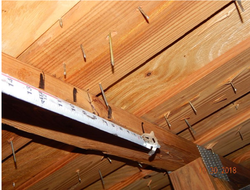
Plywood Over Battens
