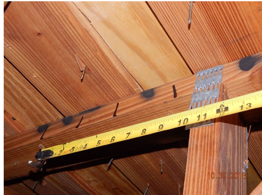
Plywood Over Battens
