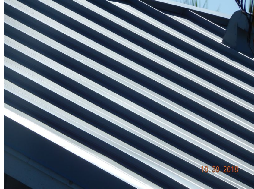
Metal Roof Covering
