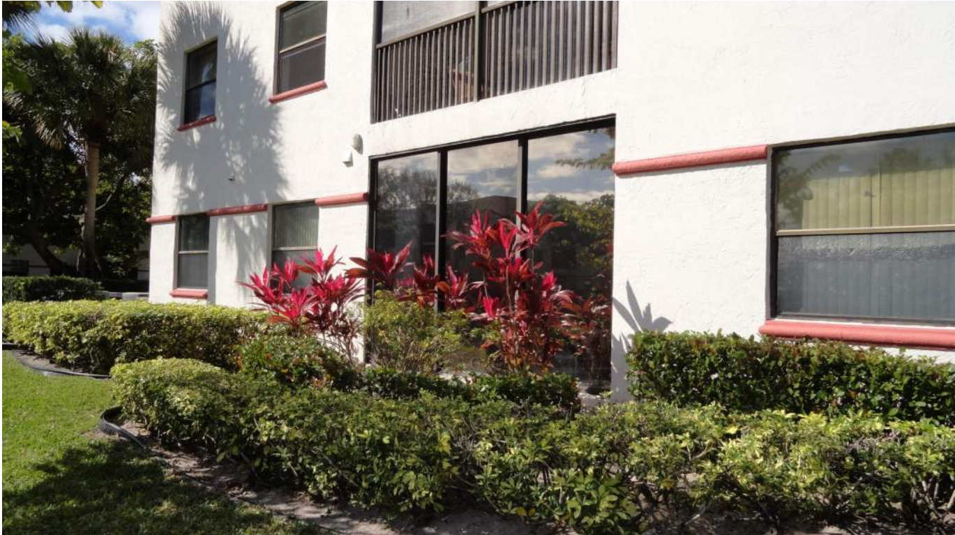
7. Opening Protection - Unprotected Unrated Glazed Entry Doors
