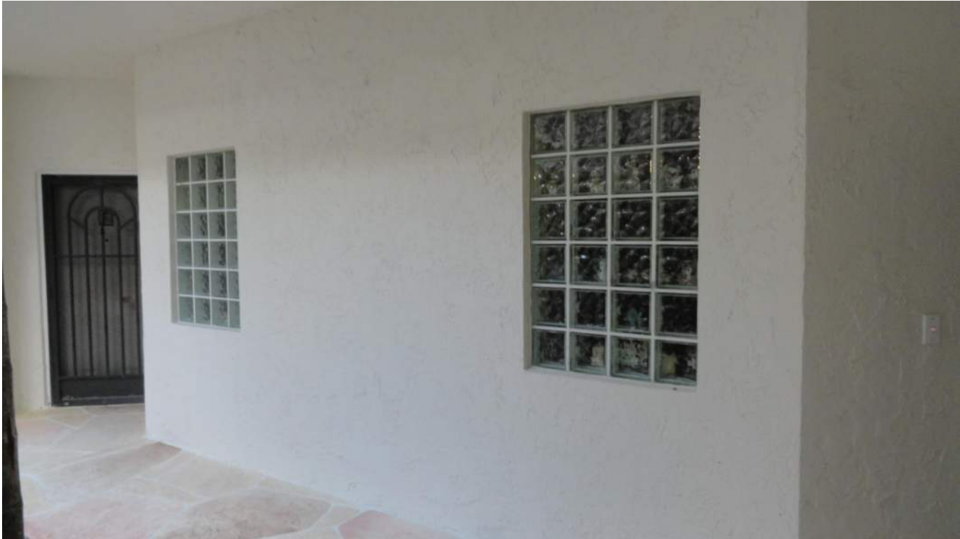
7. Opening Protection - Unprotected Unrated Glass Block Opening
