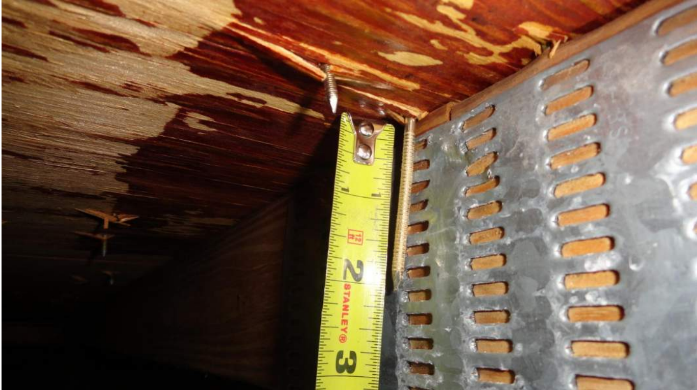
3. Roof Deck Attachment - 8d Ring Shank Nails
