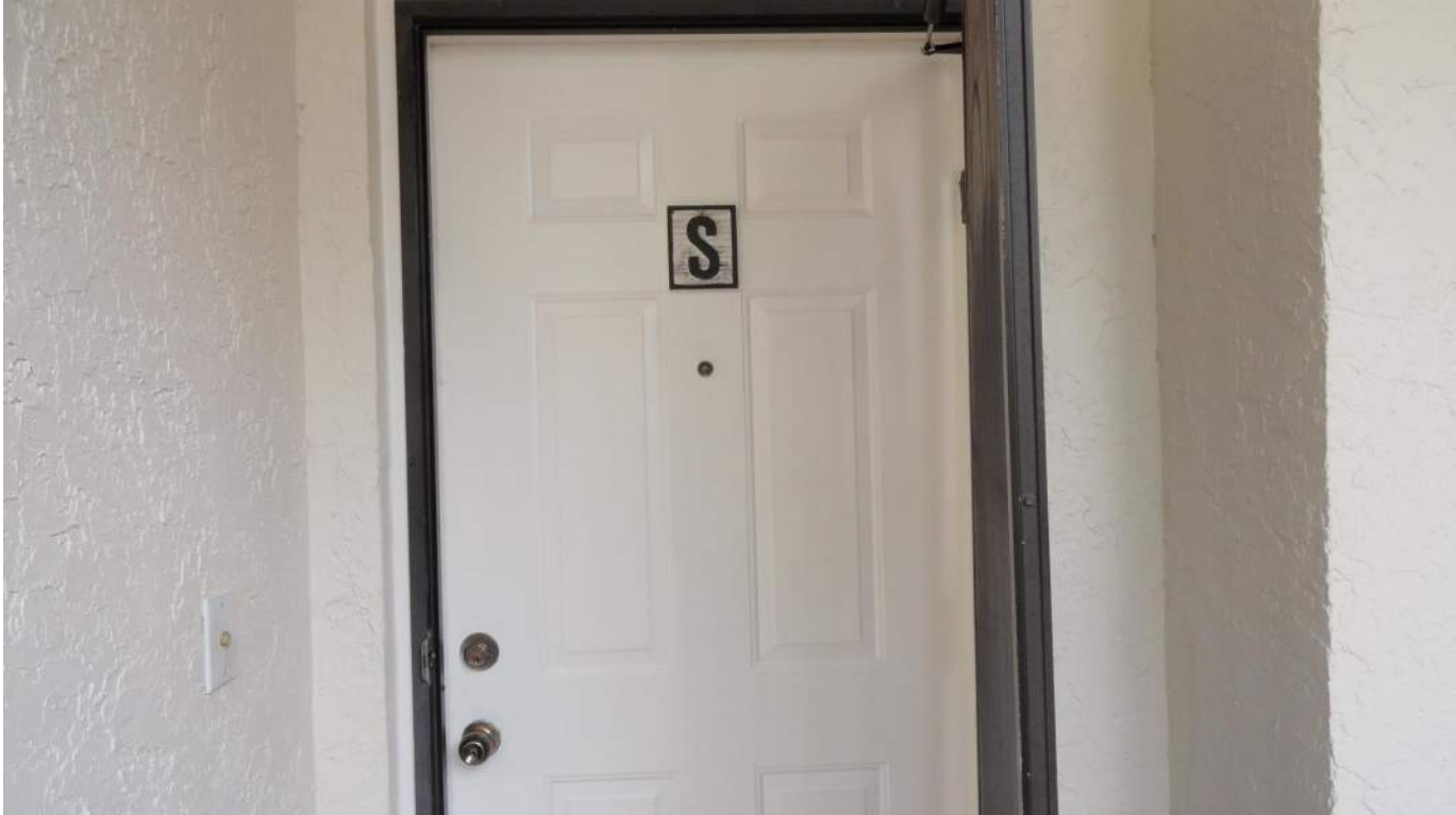
7. Opening Protection - Unprotected Unrated Unglazed Entry Doors
