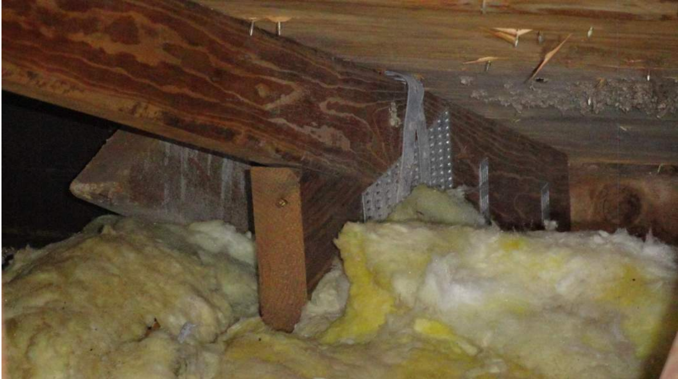
4. Roof to Wall Attachment - Double Wraps - Steel Straps Each w/ 2 Nails Min. at Face & 1 Nail Min. at Back
