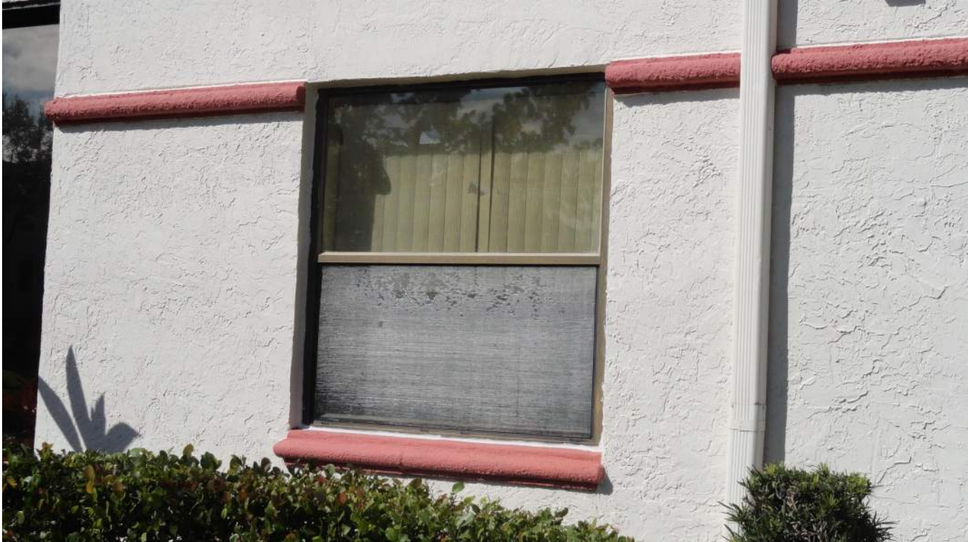
7. Opening Protection - Unprotected Unrated Windows
