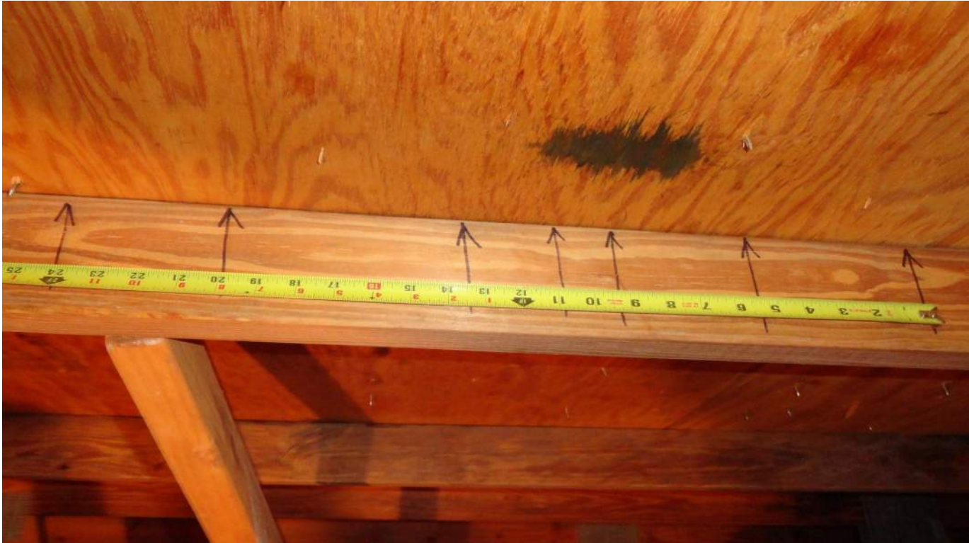
3. Roof Deck Attachment - Nails at 6" O. C. Max. in the Field
