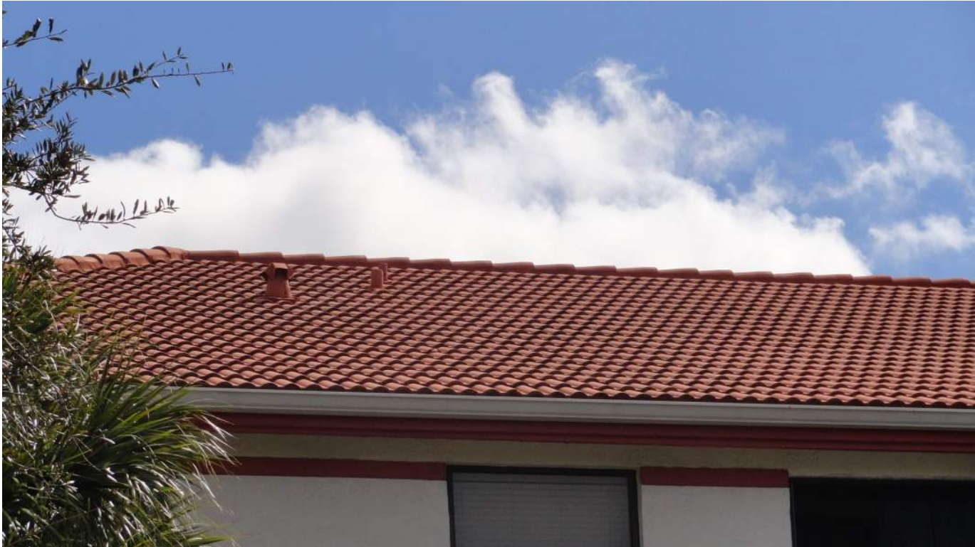
2. Roof Covering - Concrete Tile
