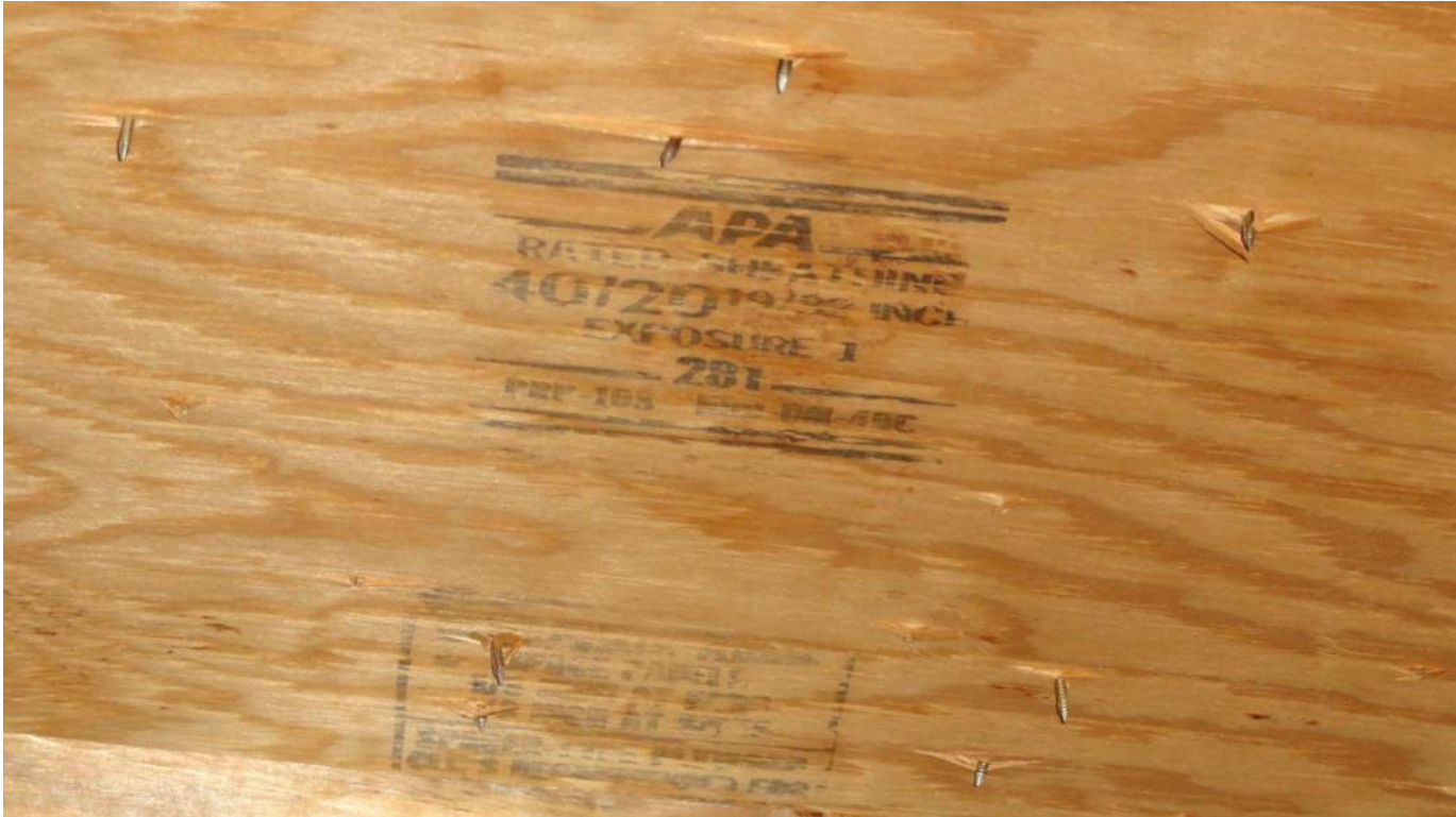
3. Roof Deck Attachment - 19/32" Plywood Deck
