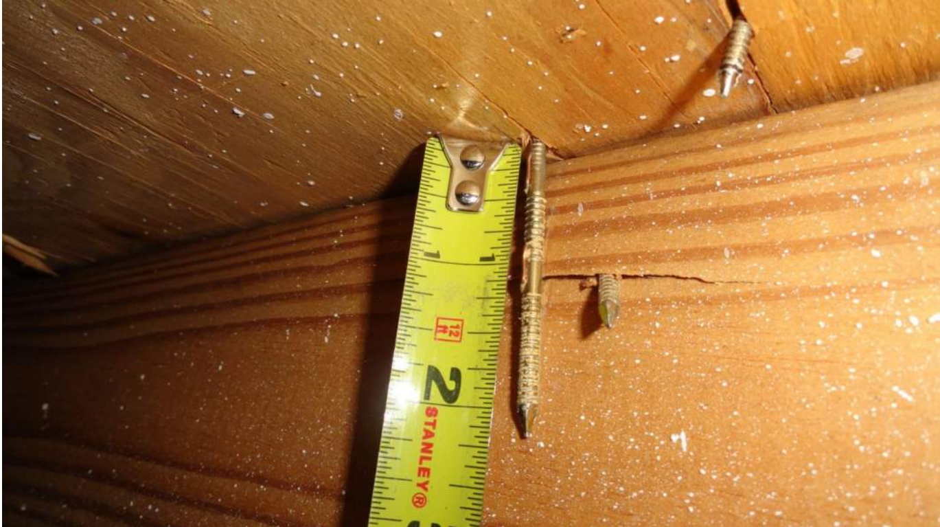
3. Roof Deck Attachment - 8d Ring Shank Nails
