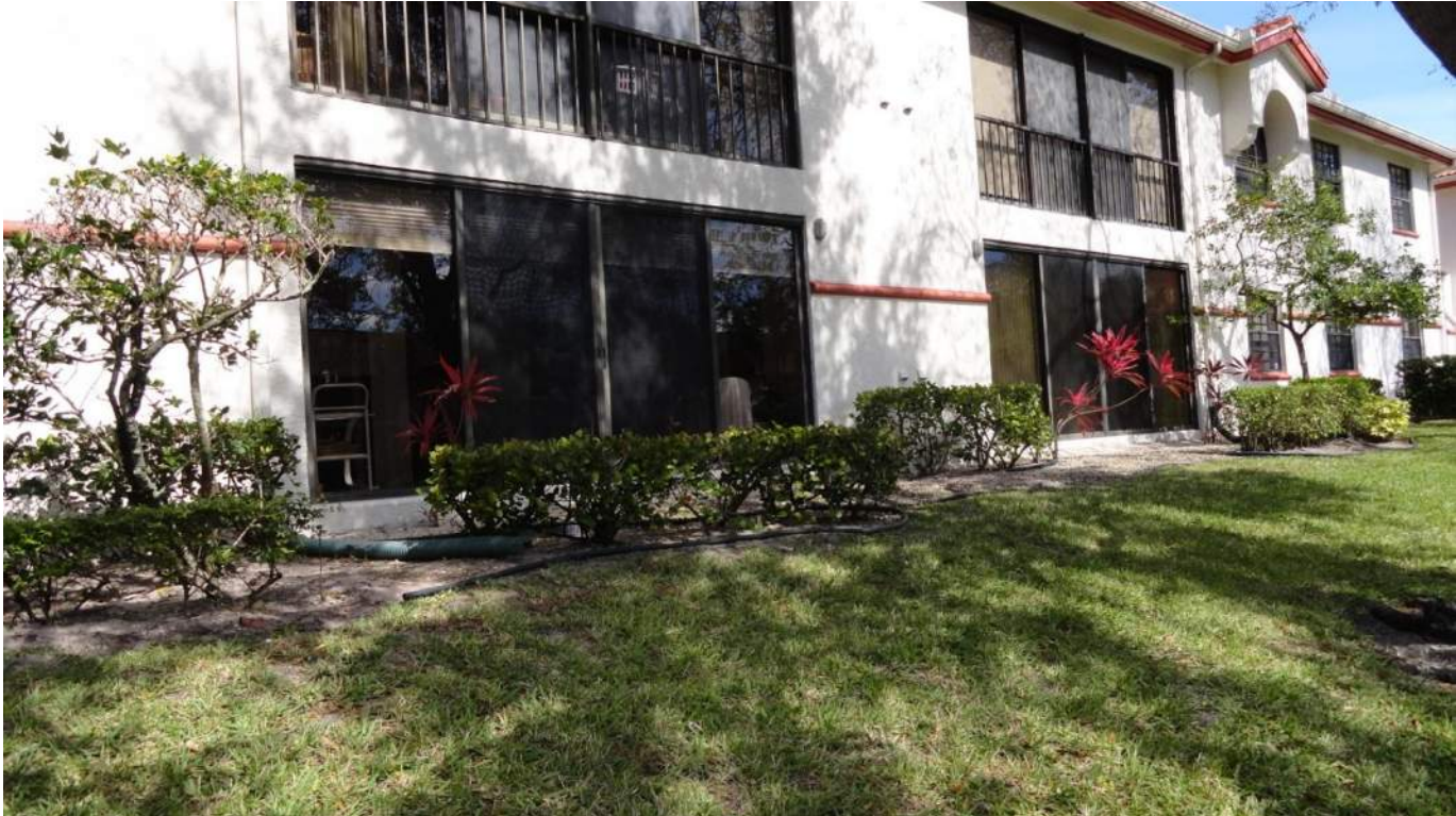
7. Opening Protection - Unprotected Unrated Glazed Entry Doors
