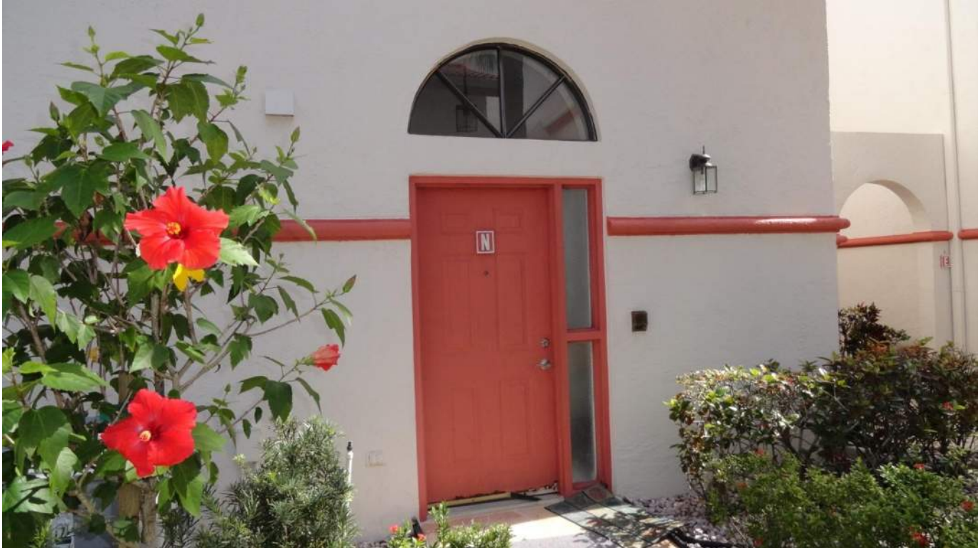
7. Opening Protection - Unprotected Unrated Unglazed Entry Doors
