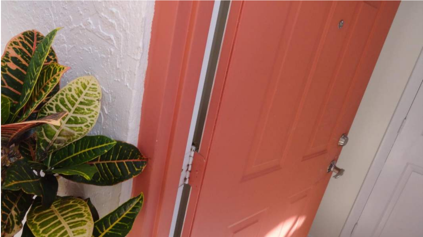
7. Opening Protection - Unprotected Unrated Unglazed Entry Doors
