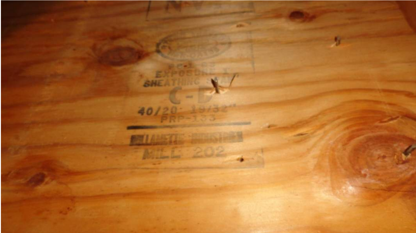
3. Roof Deck Attachment - 19/32" Plywood Deck
