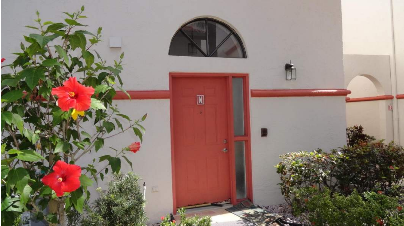
7. Opening Protection - Unprotected Unrated Unglazed Entry Doors
