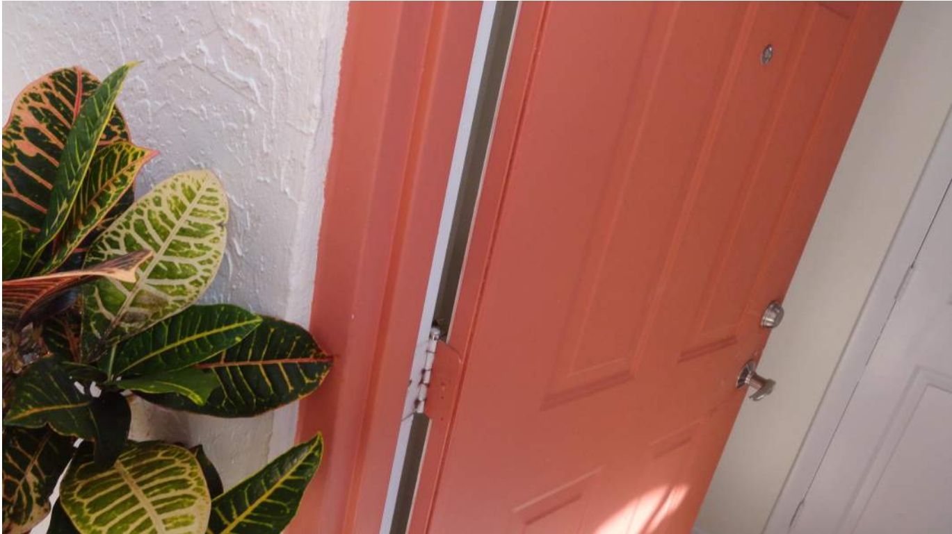
7. Opening Protection - Unprotected Unrated Unglazed Entry Doors
