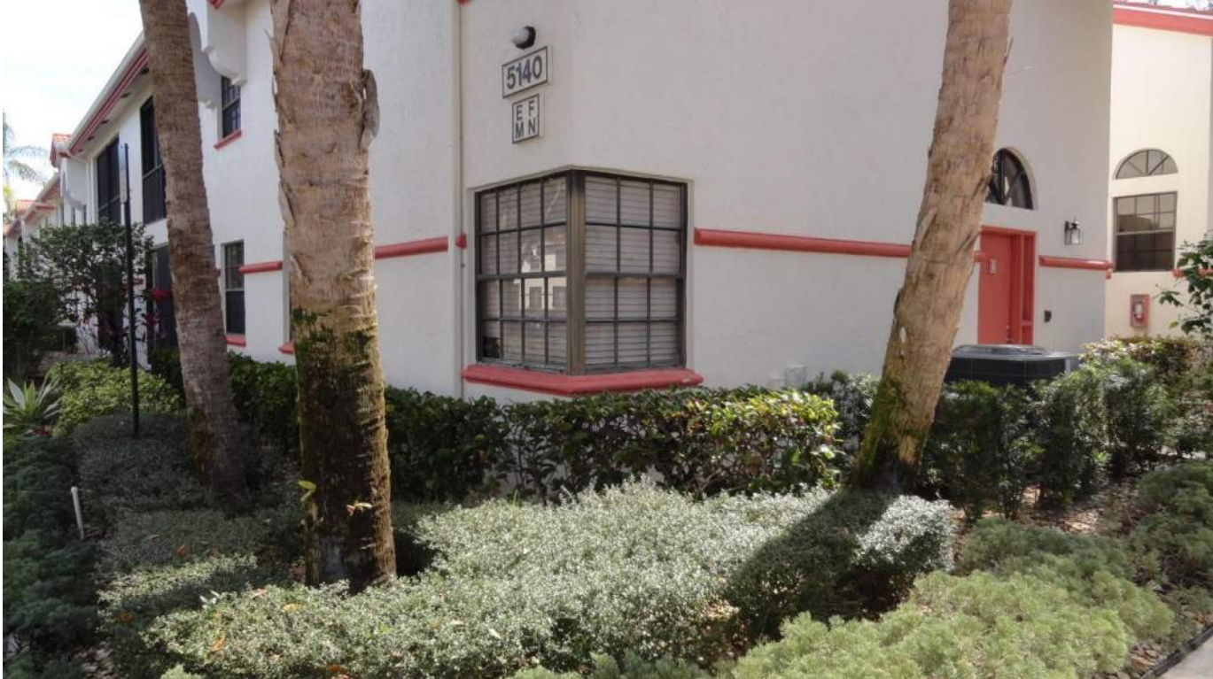
7. Opening Protection - Unprotected Unrated Windows
