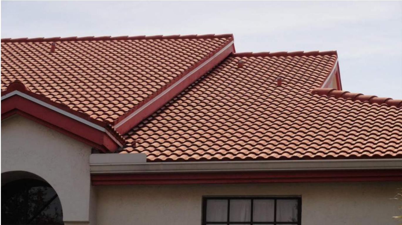
2. Roof Covering - Concrete Tile
