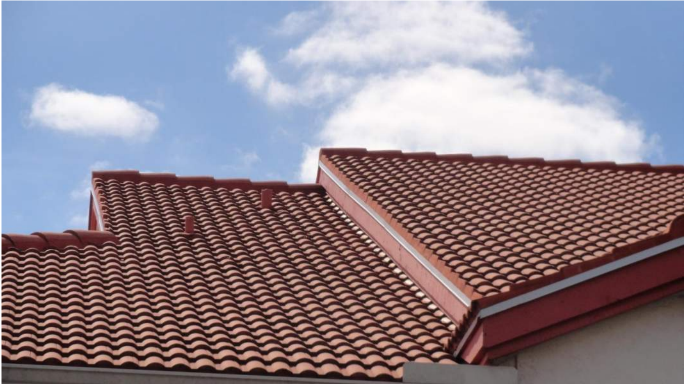
2. Roof Covering - Concrete Tile
