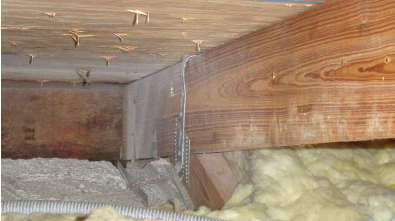
4. Roof to Wall Attachment - Single Wraps - Steel Straps w/ 2 Nails Min. at Face
