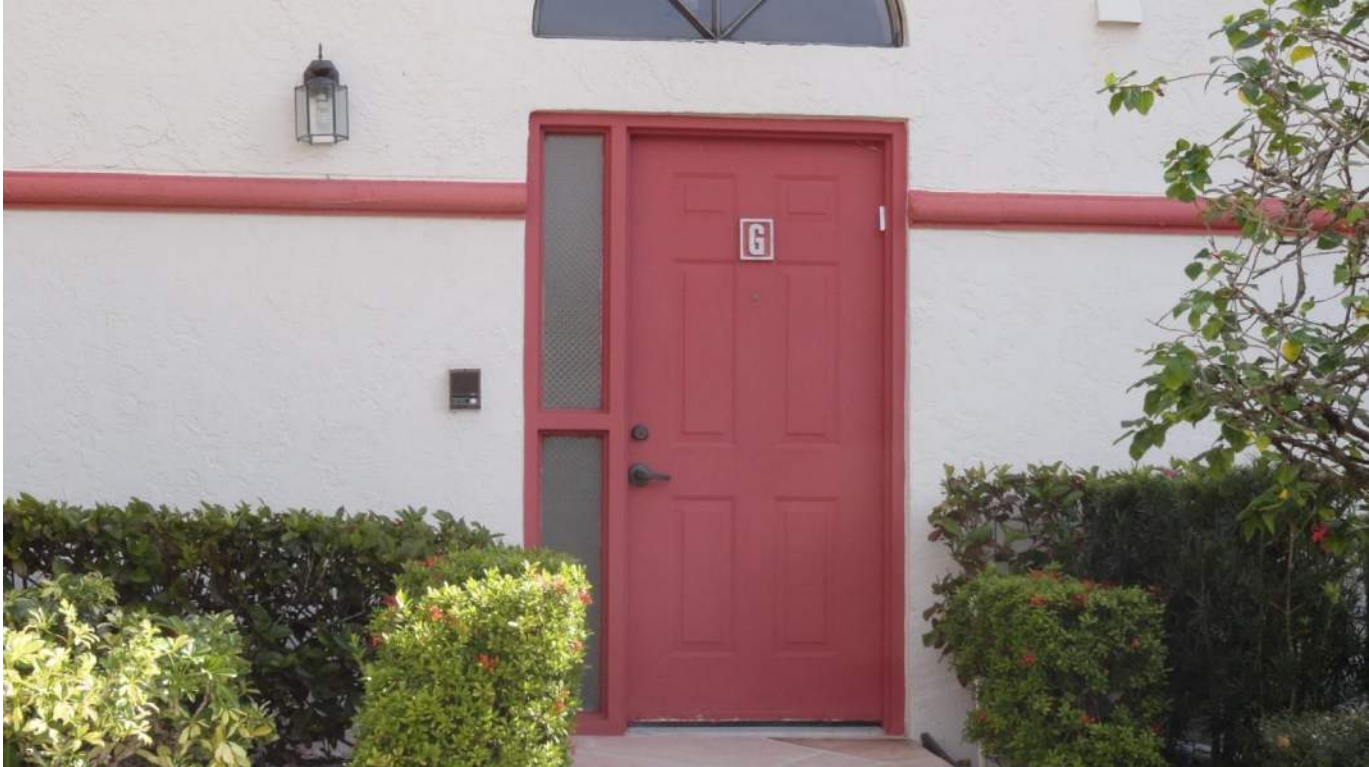
7. Opening Protection - Unprotected Unrated Unglazed Entry Doors
