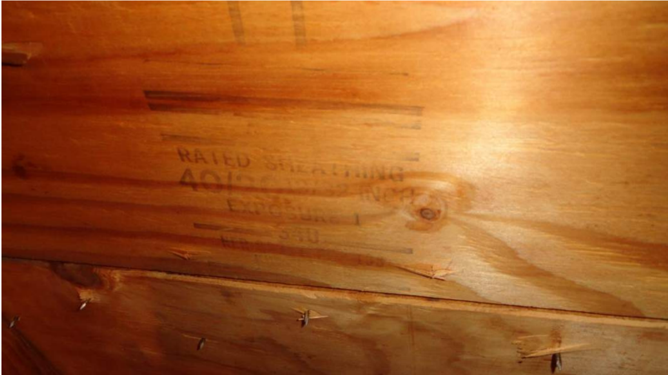
3. Roof Deck Attachment - 19/32" Plywood Deck
