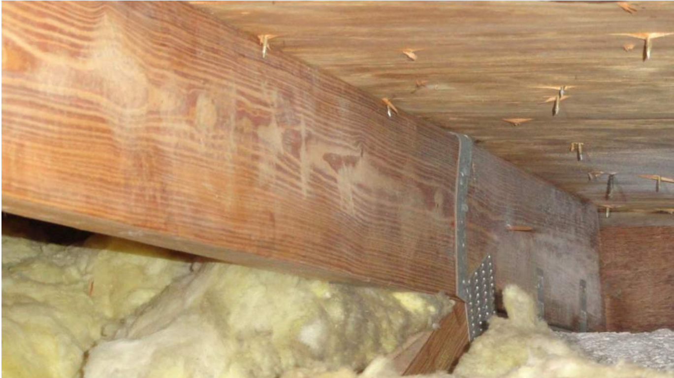
4. Roof to Wall Attachment - Single Wraps - Steel Straps w/ 1 Nail Min. at Back
