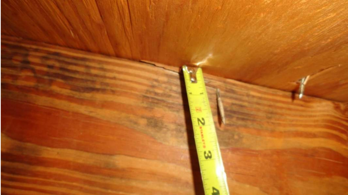
3. Roof Deck Attachment - 8d Ring Shank Nails
