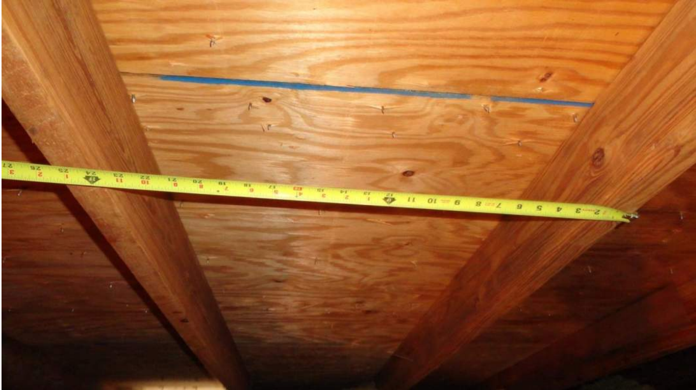
3. Roof Deck Attachment - Trusses at 24" O. C. Max.
