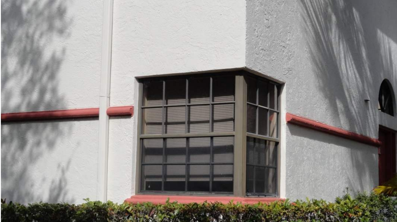
7. Opening Protection - Unprotected Unrated Windows
