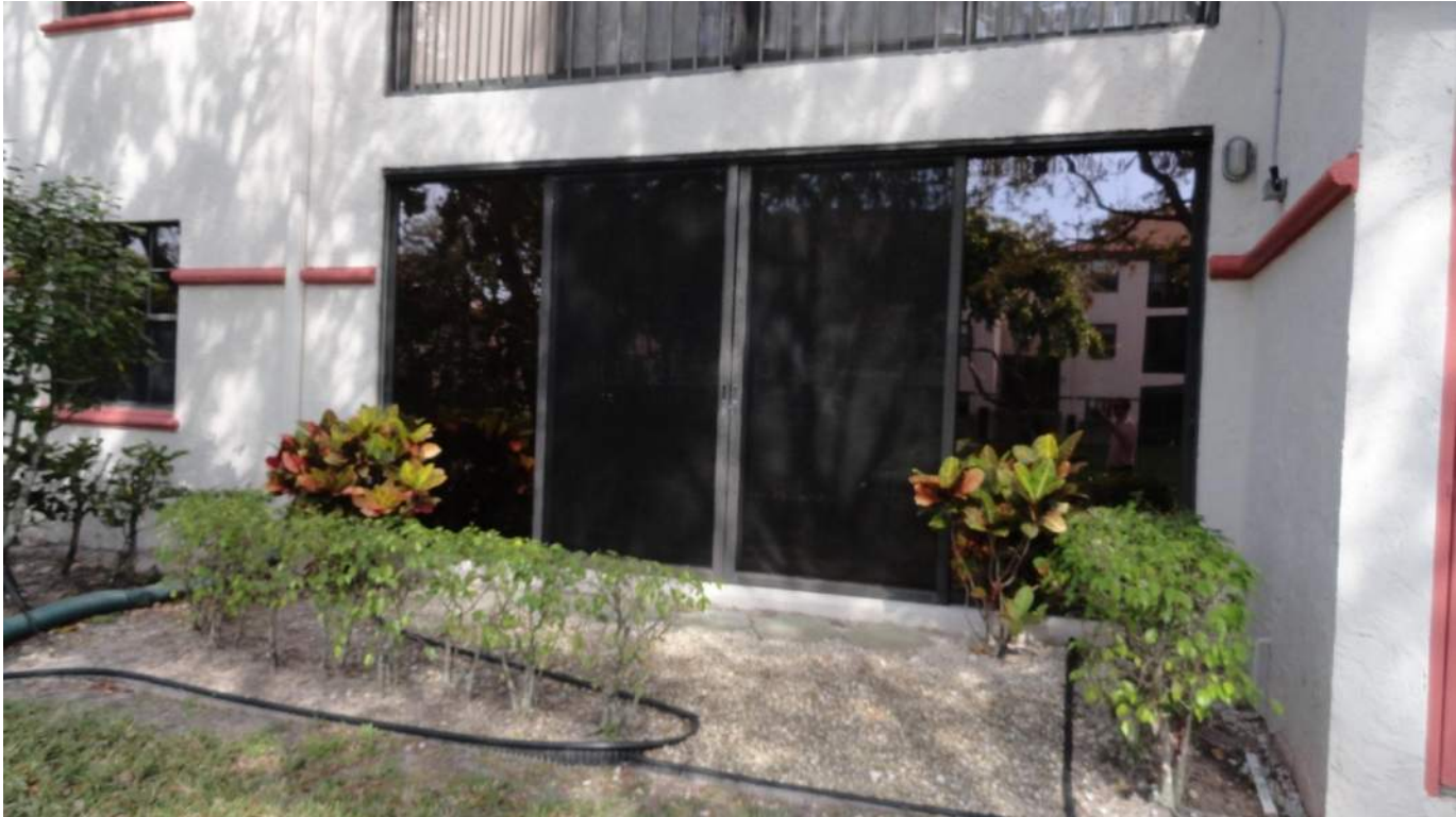
7. Opening Protection - Unprotected Unrated Glazed Entry Doors
